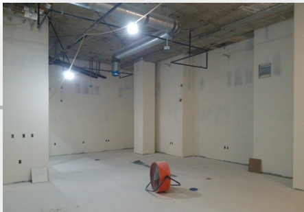
10th Floor Buildout [Construction]
