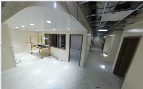
10th Floor Buildout [Construction]
