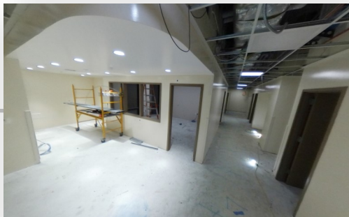
10th Floor Buildout [Construction]
