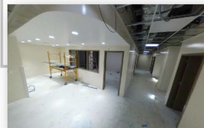
10th Floor Buildout [Construction]
