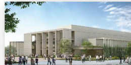
New Science, Engineering and Mathematics Building [Construction]
