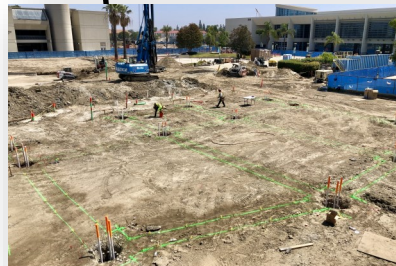
New Veterans' Resource Center & Student Activities Center Expansion [Construction]
