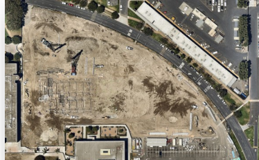
New Science, Engineering and Mathematics Building [Construction]
