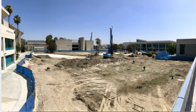
Veterans' Memorial Bridge, Plaza, & Tribute Garden [Construction]
