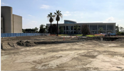
Veterans' Memorial Bridge, Plaza, & Tribute Garden [Construction]
