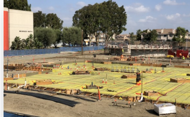
New Science, Engineering and Mathematics Building [Construction]
