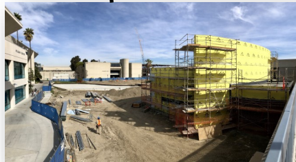
New Veterans' Resource Center & Student Activities Center Expansion [Construction]
