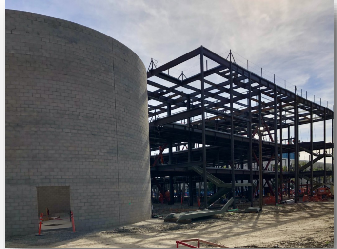
New SEM Construction Progress—February 5, 2020
