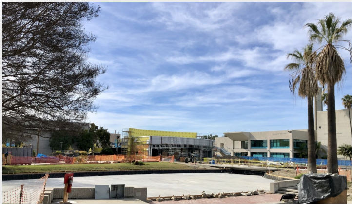
VRC/SAC Construction Progress—February 5, 2020
