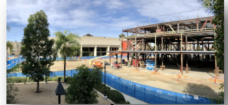
New Science, Engineering and Mathematics Building [Construction]
