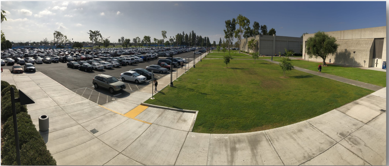
Completed Parking Lot 5 Realignment from the LLRC at Cypress College
