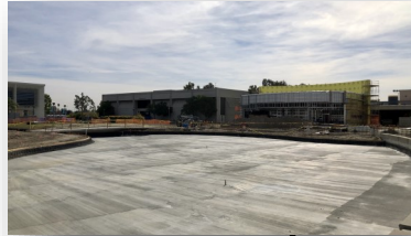
Veterans' Memorial Bridge & Tribute Garden [Construction]
