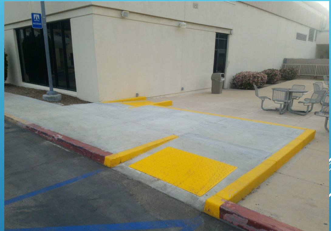
Drop off Circle ADA Ramp
