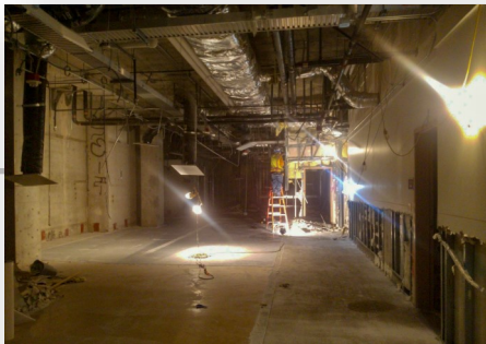
10th Floor Buildout [Construction]
