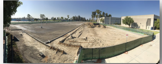
Swing Space Projects Parking Lot #5 [Construction]
