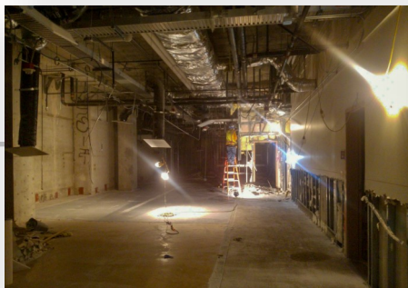
10th Floor Buildout [Construction]
