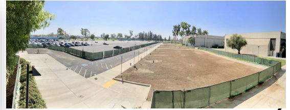
Swing Space Projects Parking Lot #5 [Close-Out]
