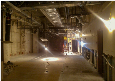
10th Floor Buildout [Construction]
