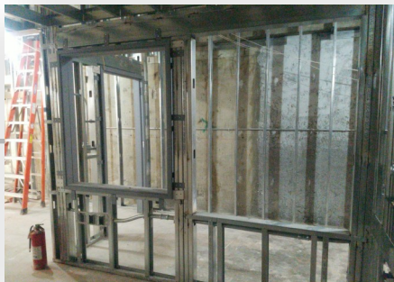
10th Floor Buildout [Construction]
