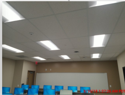
7th Floor Buildout [Complete]
