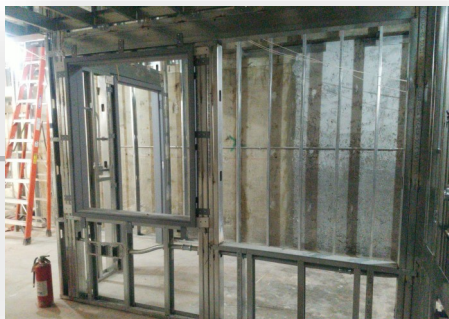
10th Floor Buildout [Construction]
