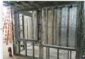
10th Floor Buildout [Construction]
