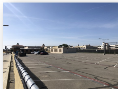
Central Plant Replacement and Expansion [Construction]
