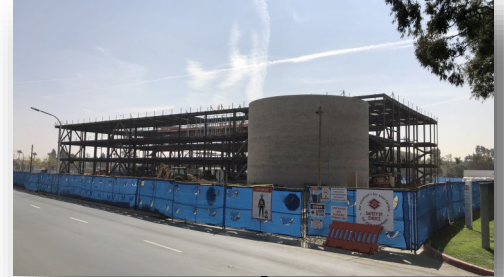
New Science, Engineering and Mathematics Building [Construction]
