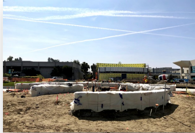
Veterans' Memorial Bridge, Plaza, & Tribute Garden [Construction]
