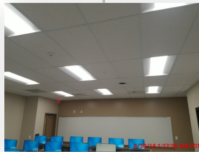
7th Floor Buildout [Close-Out]
