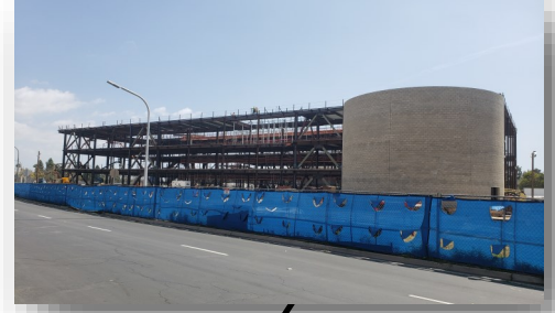
New Science, Engineering and Mathematics Building [Construction]
