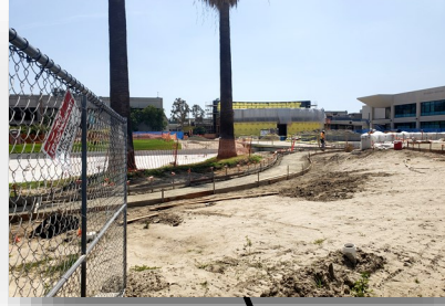
Veterans' Memorial Bridge, Plaza, & Tribute Garden [Construction]
