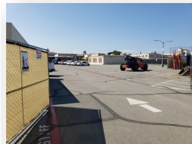
Central Plant Replacement and Expansion [Construction]
