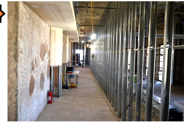
Anaheim Campus—7th Floor Buildout Construction Progress February 2018
