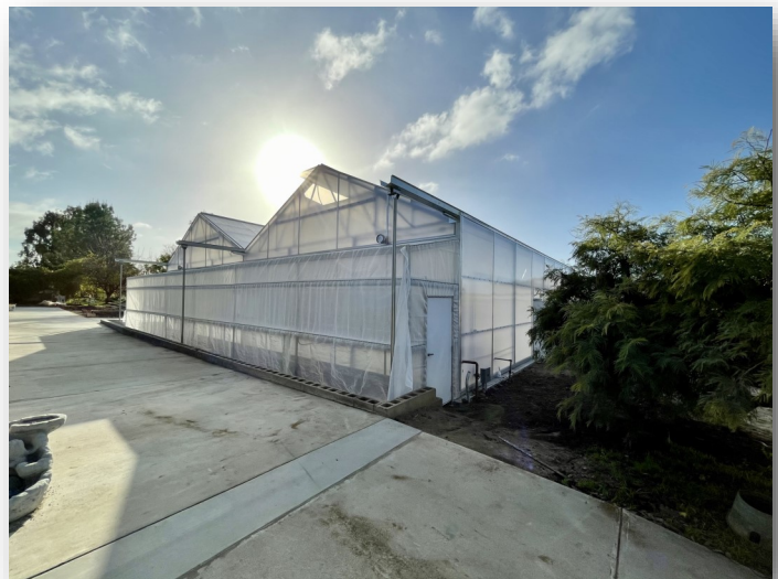
Greenhouse Replacement Construction Progress — March 2021
