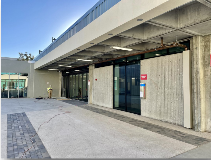
SAC Construction Progress — March 2021
