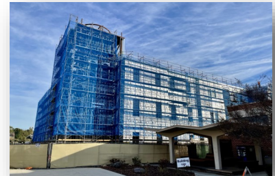
New Instructional Building [Construction]
