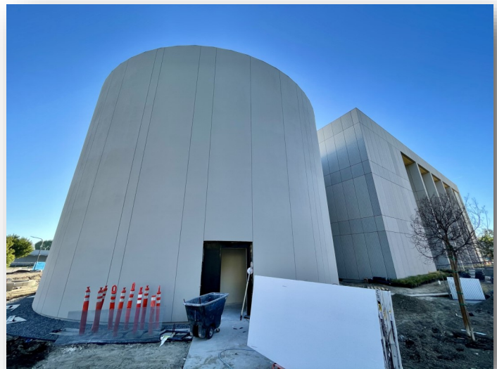
New SEM's IDC Construction Progress —March 2021
