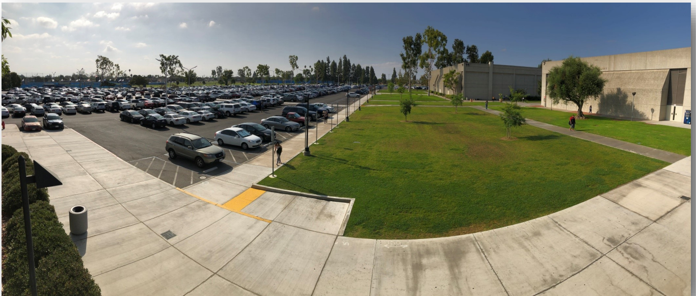
Completed Parking Lot 5 Realignment from the Library & Learning Resource Center (LLRC) at Cypress College
