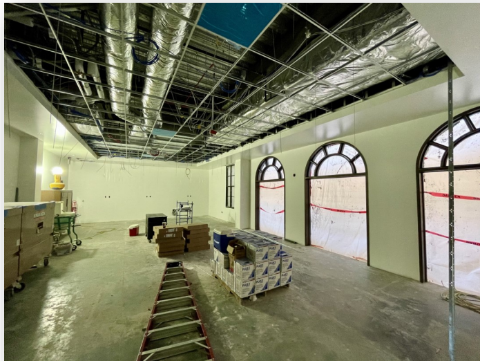
New Instructional Interior Construction Progress — March 2021
