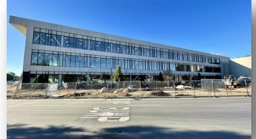
New Science, Engineering and Mathematics Building [Construction]
