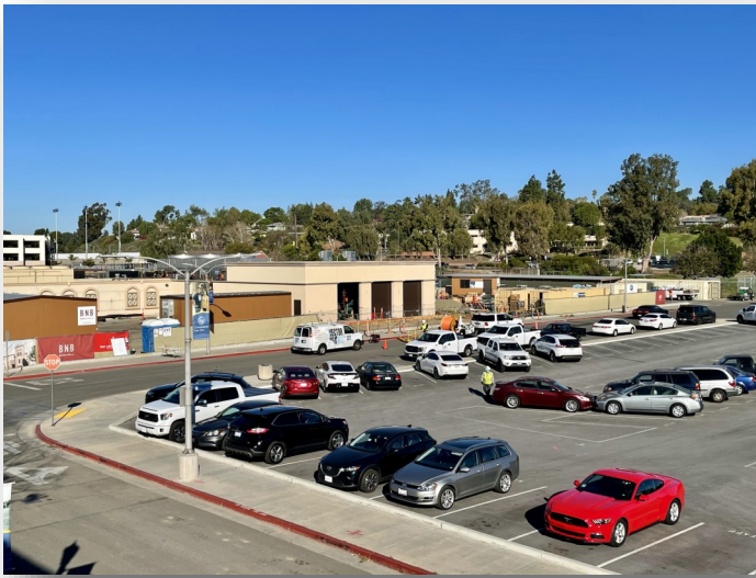
Central Plant Construction Progress —March 2021
