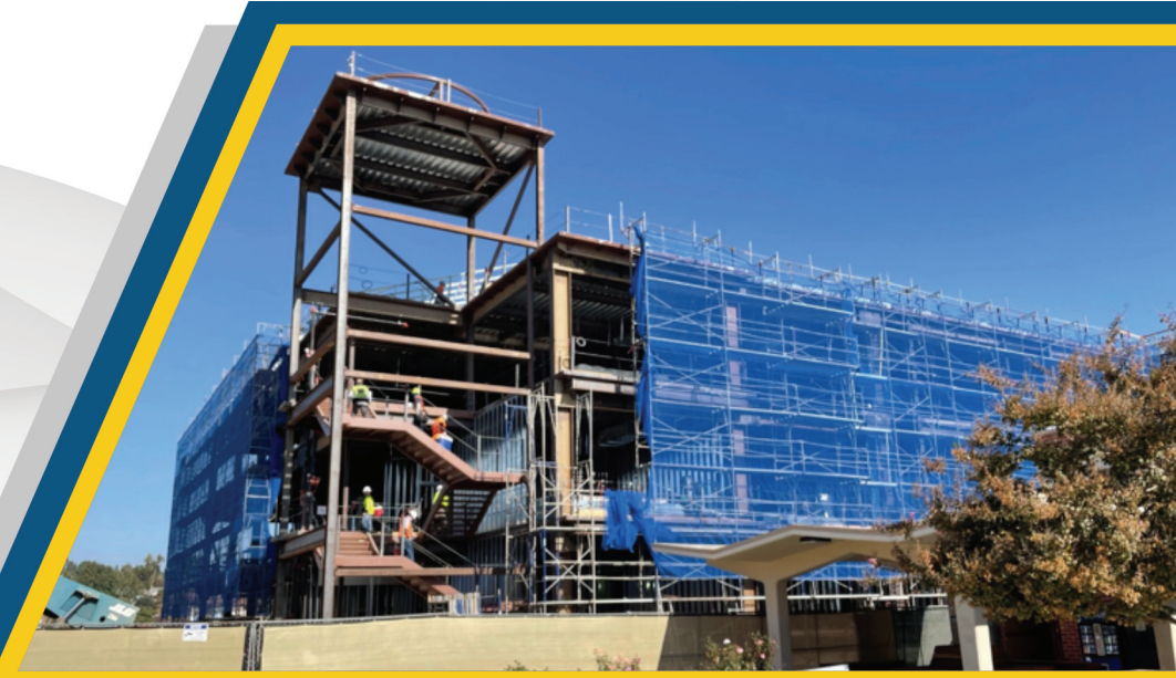
Fullerton College Construction Progress New Instructional Building
