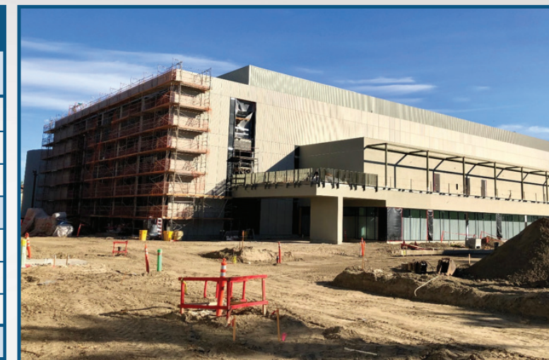
Cypress College Construction Progress New SEM
