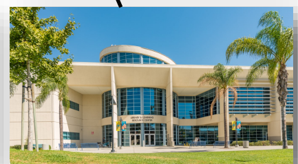
LLRC Secondary Data Center (Phase II) [ Implementation ]
