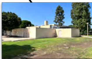
Wilshire Chiller Plant Relocation [DSA Review]
