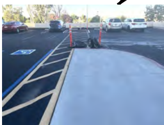
Anaheim Campus Tower First Floor Life/Safety Renovation [DSA Review]
