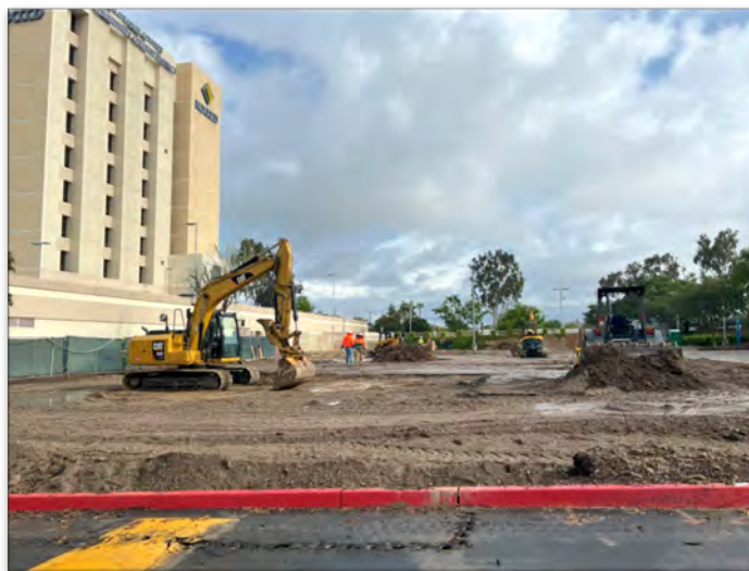
Swing Space / Interim Housing—Demolition of the Playground
