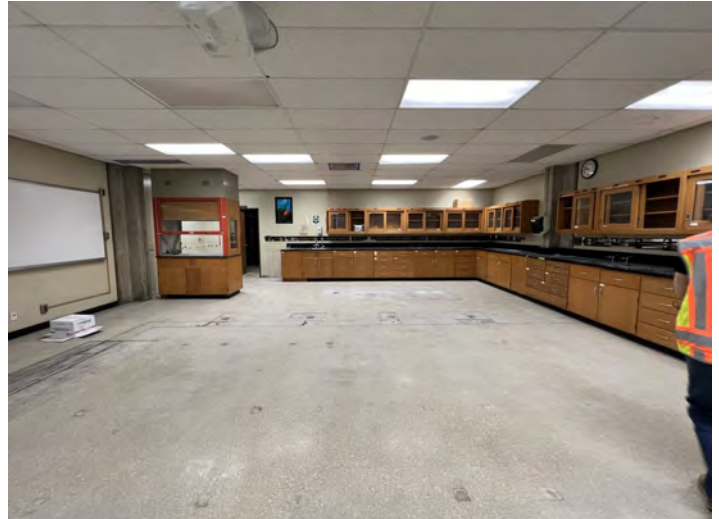
Swing Space—Fine Arts—Construction Activities
