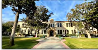
Renovate Building 300 [DSA Review]
