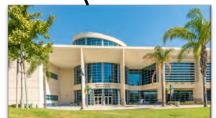
LLRC Secondary Data Center (Phase II) [Close-Out]
