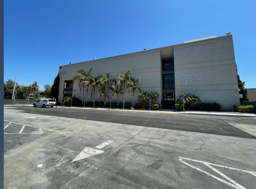
Americans with Disabilities Act (ADA) Barrier Removal – Parking Lot 1
