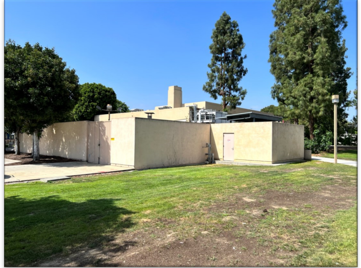
Wilshire Chiller Plant Relocation — Exterior Facade
