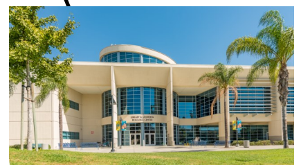
LLRC Secondary Data Center (Phase II) [Close-out]
