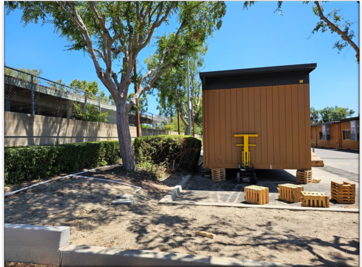
Swing Space / Interim Housing—Modular Building Construction Activities
