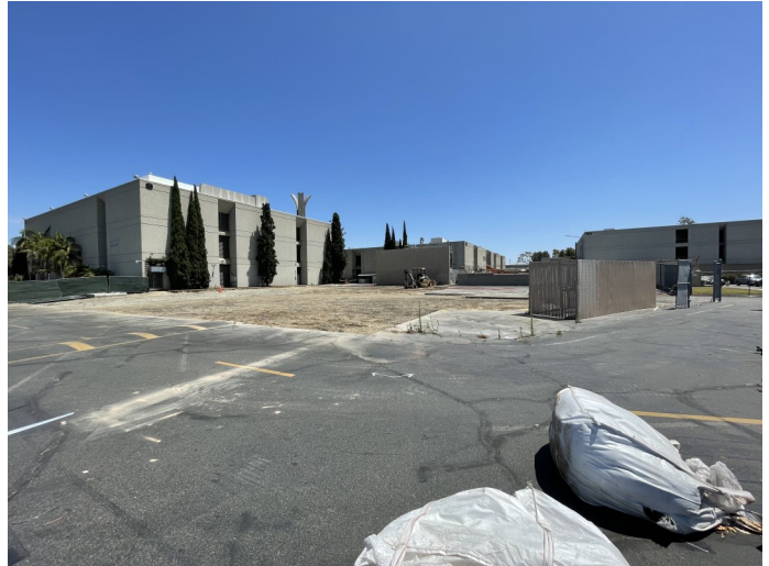
Swing Space-HRC: Kitchen, Dining, and Bathroom Construction Activities
