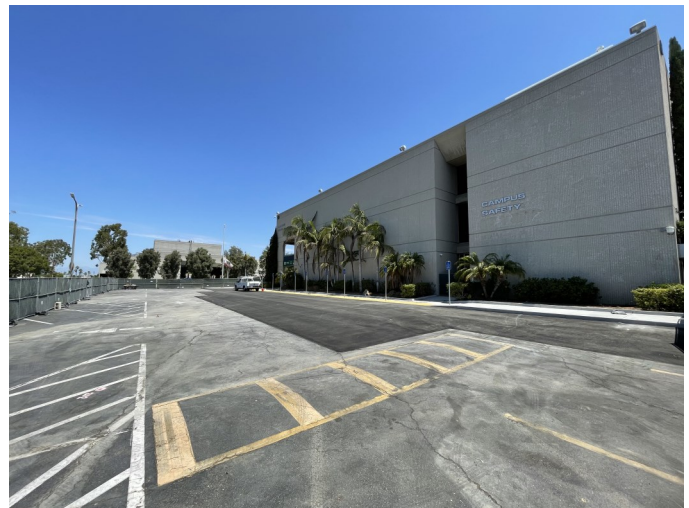
Swing Space-HRC: Parking Lot 1 Construction Activities
