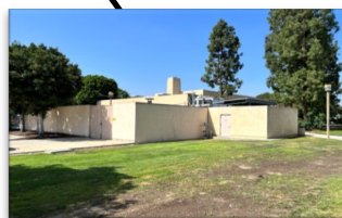
Wilshire Chiller Plant Relocation [DSA Review]
