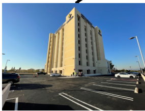
Anaheim Campus Tower First Floor Life/Safety Renovation [Bidding]
