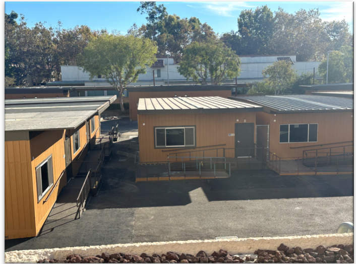
Swing Space / Interim Housing—Modular Building Construction Activities
