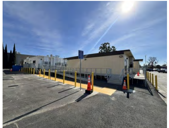
Swing Space—HRC Kitchen, Restroom and Dining Room — Modular Building Construction Activities
