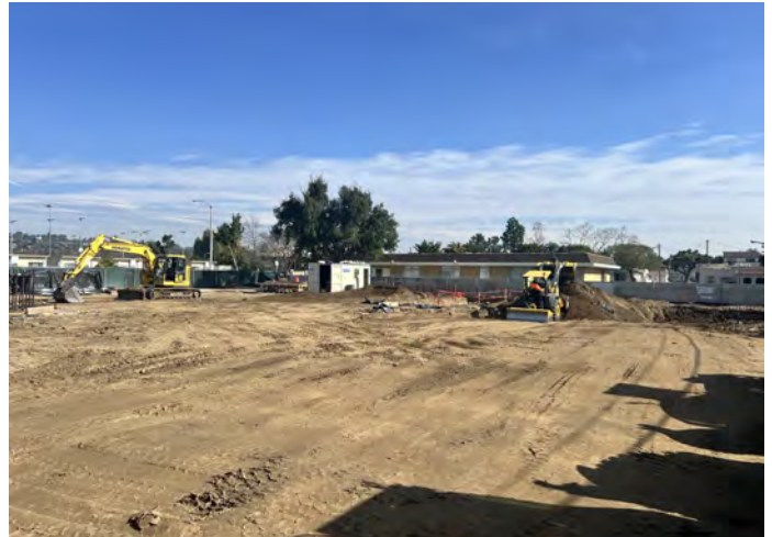
Chapman/Newell Instruction Building— Construction Activities
