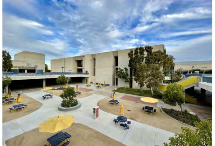
Fine Arts Building Renovation— Current View
