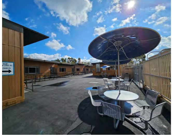
Swing Space — Interim Housing — Completed Construction
