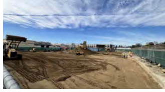
New Maintenance & Operations Building [Construction]
