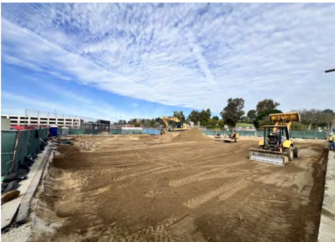
New M&O Building - Construction Activities
