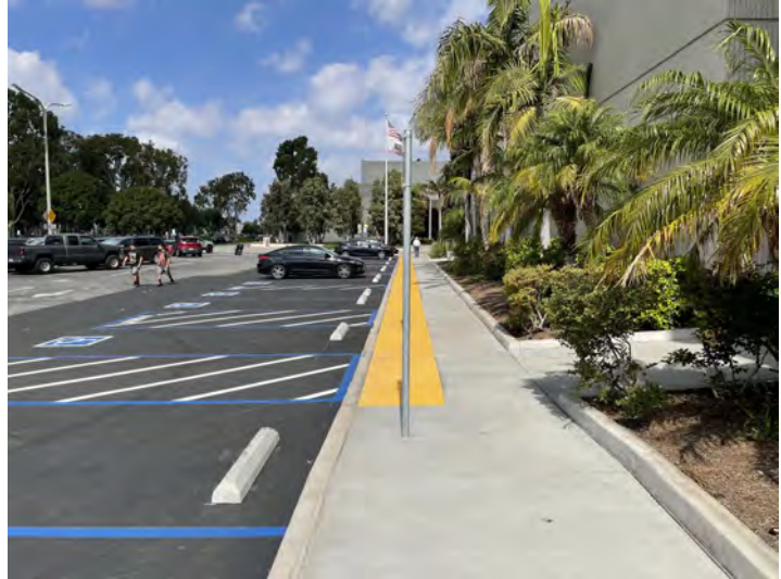
Swing Space—Hotel, Restaurant, and Culinary Arts: Americans with Disabilities Act (ADA) Parking Lot 1— Completed Construction
