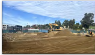
New Maintenance & Operations Building [Construction]
