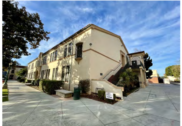
Renovate Building 300 - Exterior Elevation
