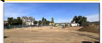
Chapman / Newell Instructional Building [Construction]
