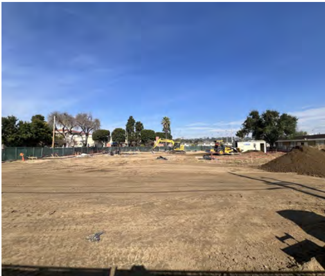
Chapman / Newell Instructional Building -- Construction Activities
