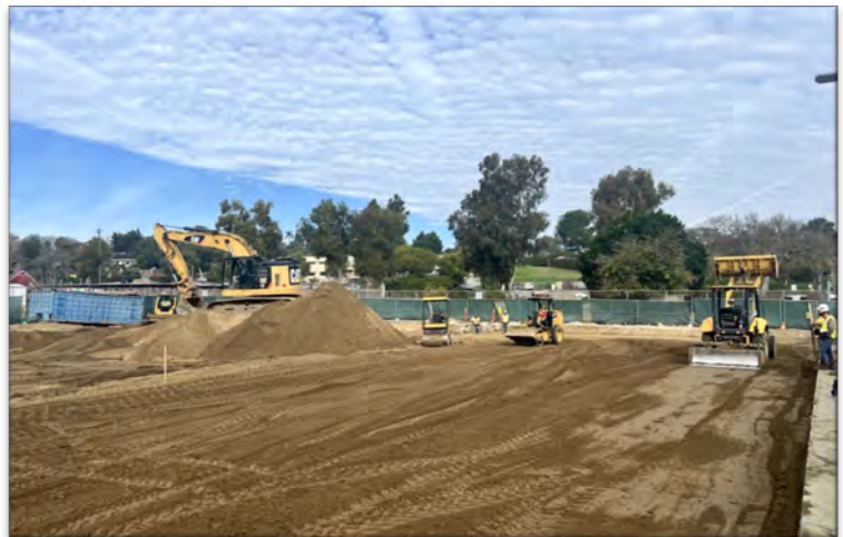
New M&O Building - Construction Activities
