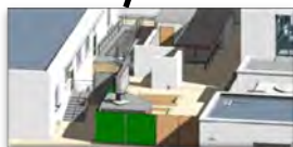
Wilshire Chiller Plant Relocation [Bidding]
