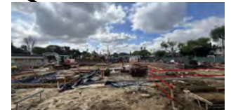
Chapman/Newell Instructional Building [Construction]
