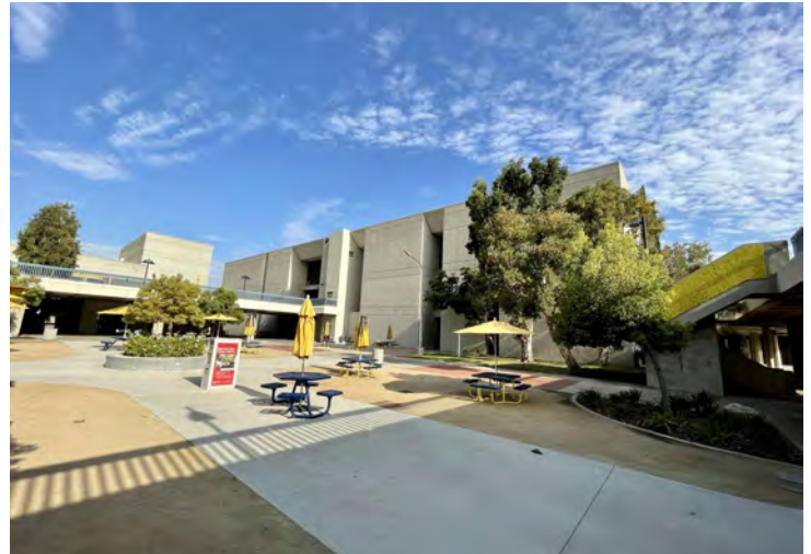
Fine Arts Building Renovation — Exterior
