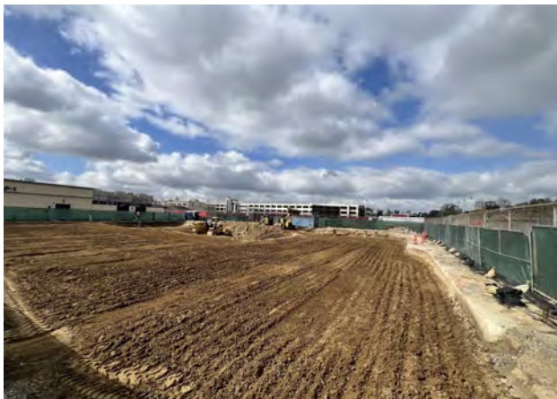
New M&O Building - Foundation Construction Activities
