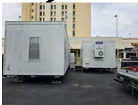
Anaheim Tower First Floor Life/ Safety Renovation [Construction]
