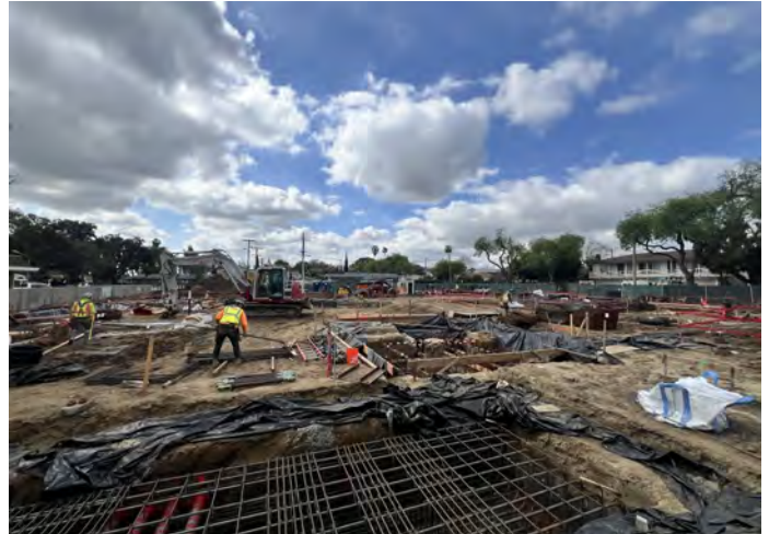
Chapman/Newell Instruction Building — Foundation Grade Beams Construction Activities
