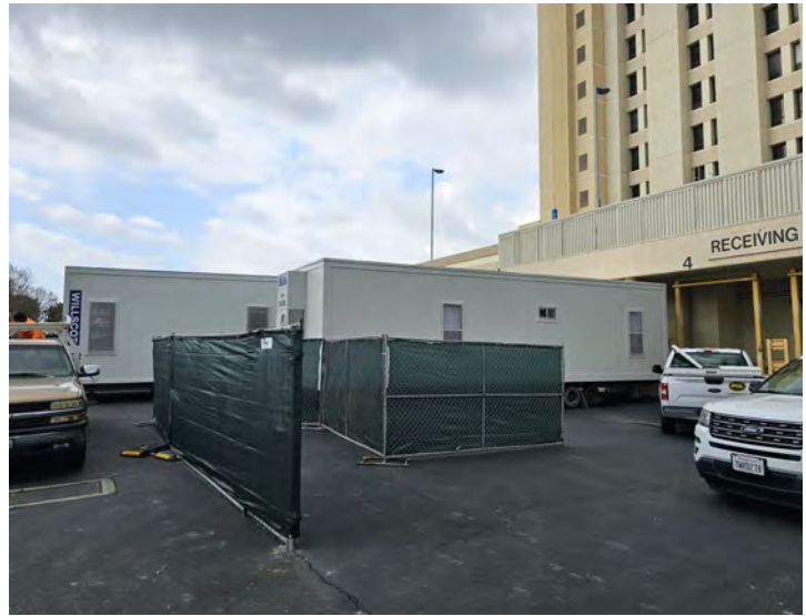
Anaheim Campus Tower First Floor Life/Safety Renovation: Construction Activities
