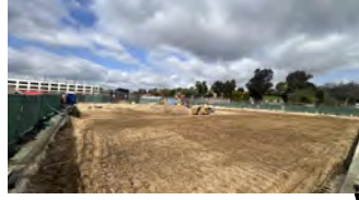
New Maintenance & Operations Building [Construction]
