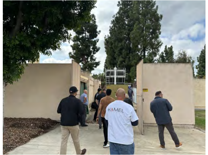
Wilshire Chiller Plant Relocation — Job walk with prequalified bidders and associated subcontractors
