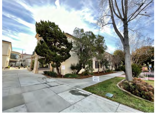
Renovate Building 300 - Exterior
