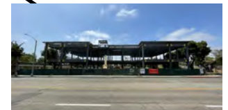
Chapman/Newell Instructional Building [Construction]
