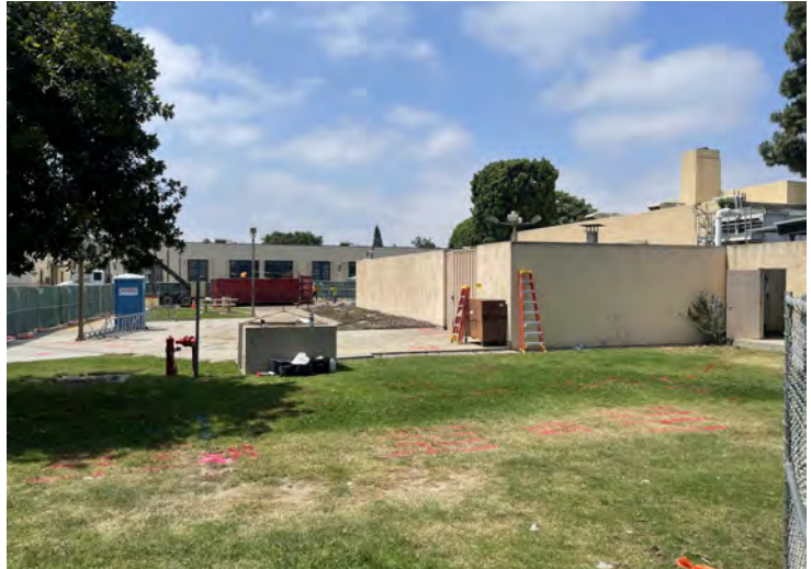
Wilshire Chiller Plant — Construction Activities
