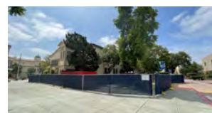
Renovate Building 300 [Construction]
