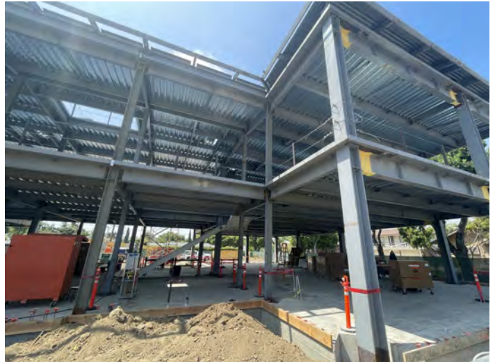
Chapman/Newell Instruction Building — Construction Activities
