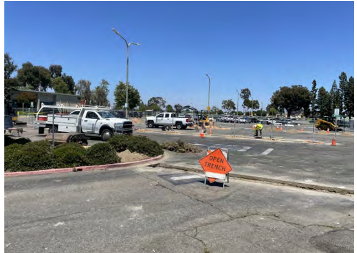
Electrical Vehicles (EV) SCE Charging Stations — Lot 4 — Construction Activities
