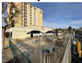
Outdoor Patio Remodel [DSA Review]
