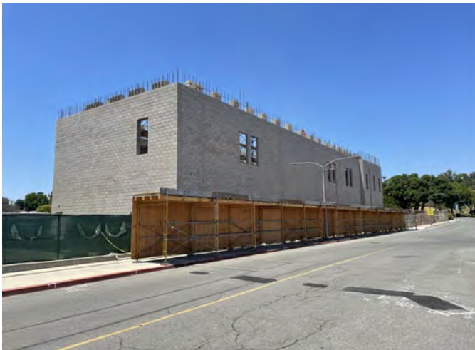
New M&O Building - Construction Activities
