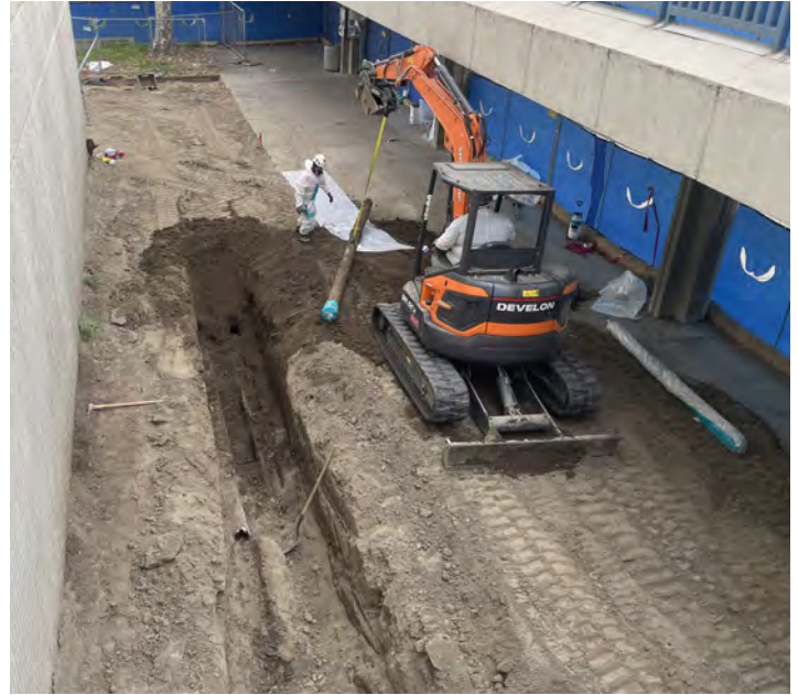
Fine Arts Building Renovation — Construction Activities
