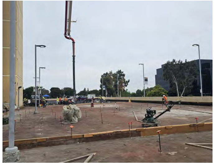
Anaheim Tower First Floor Life/Safety Renovation — Construction Activities
