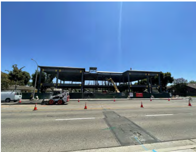
Chapman/Newell Instruction Building — Construction Activities
