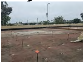
Anaheim Tower First Floor Life/ Safety Renovation [Construction]
