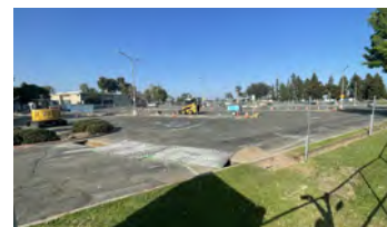
Electrical Vehicles (EV) SCE Charging Stations-Lot 4 [Construction]
