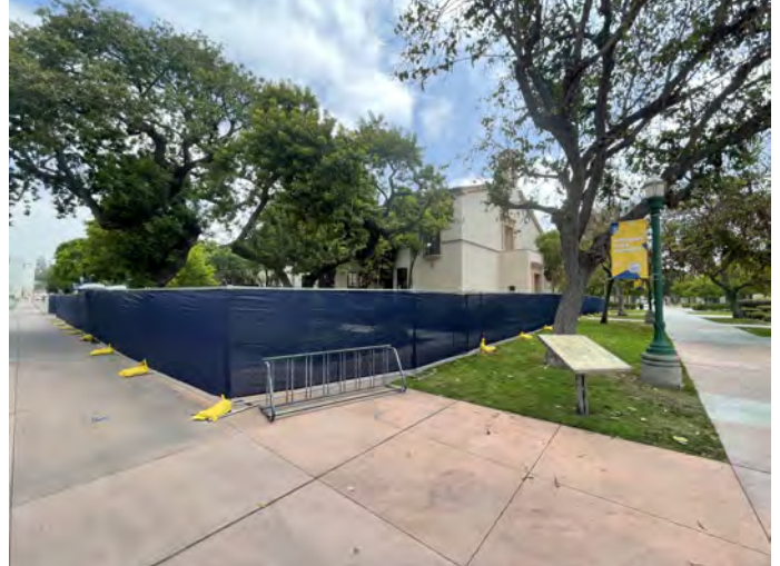
Renovate Building 300 - Exterior Building
