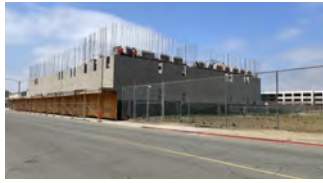
New Maintenance & Operations Building [Construction]
