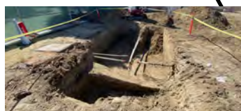
Wilshire Chiller Plant Relocation [Construction]
