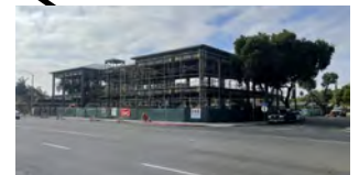
Chapman/Newell Instructional Building [Construction]
