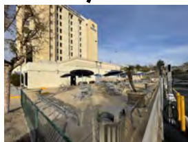
Outdoor Patio Remodel [Bidding]
