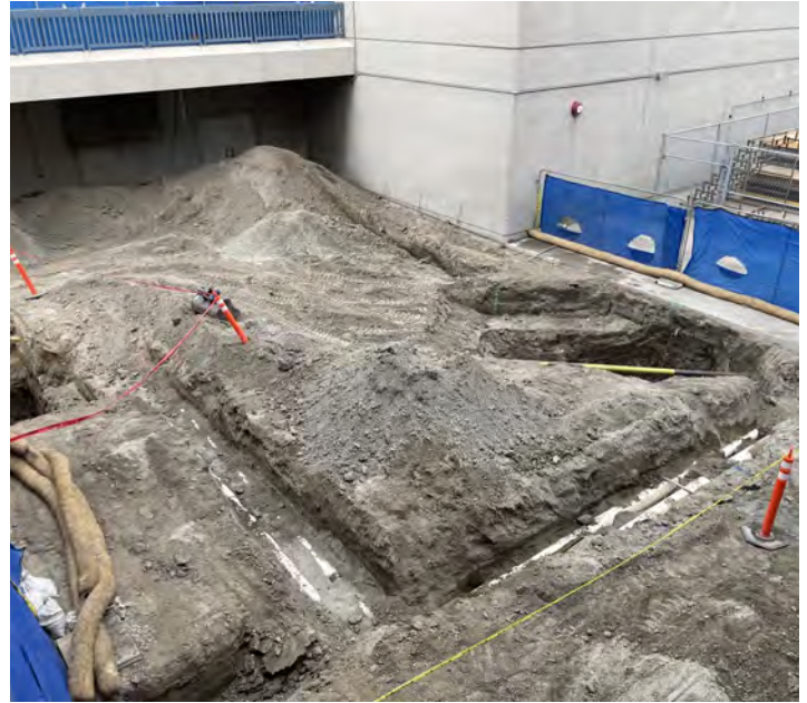
Fine Arts Building Renovation — Construction Activities
