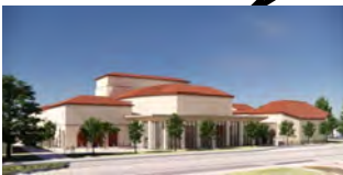
New Performing Arts Complex - Demolish Buildings 1100 and 1300 [Pre-Bidding]
