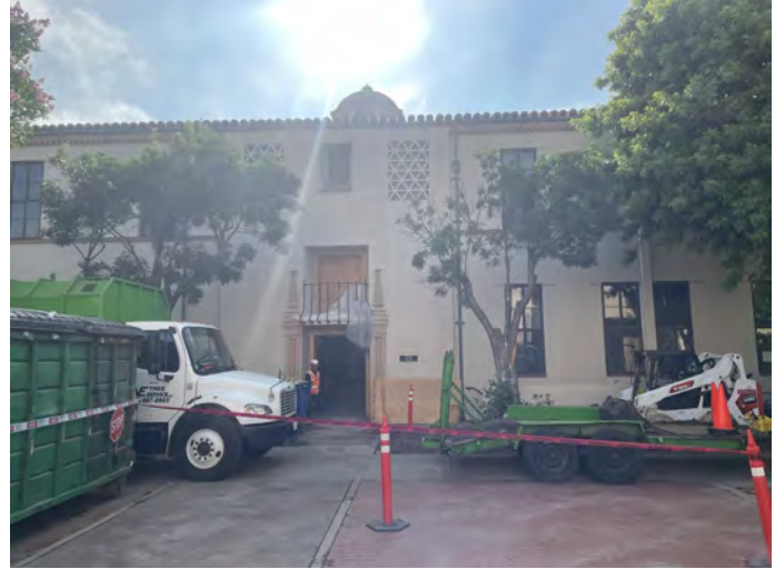
Renovate Building 300 - Construction Activities
