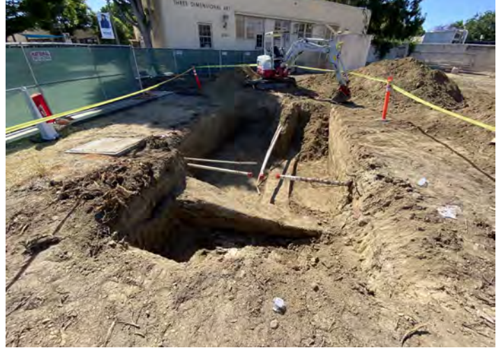
Wilshire Chiller Plant — Construction Activities
