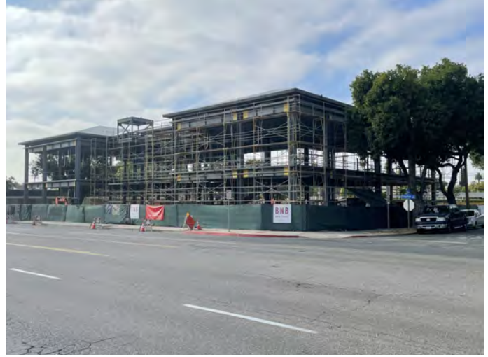
Chapman/Newell Instruction Building — Construction Activities
