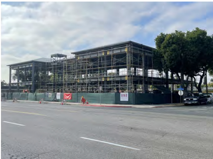
Chapman/Newell Instruction Building — Construction Activities
