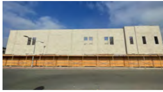
New Maintenance & Operations Building [Construction]
