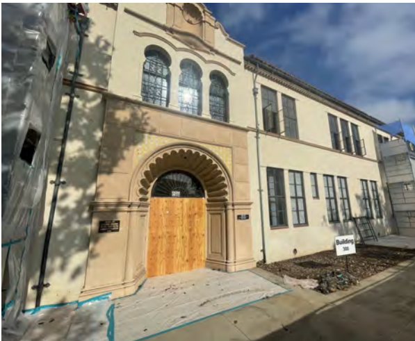
Renovate Building 300 - Construction Activities
