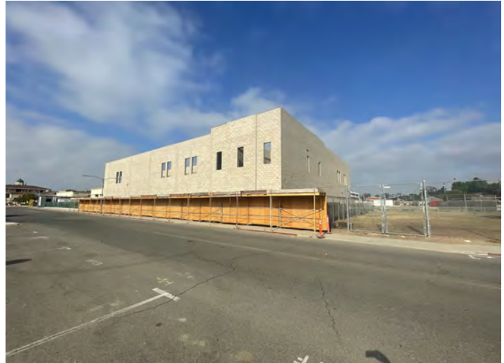
New M&O Building - Construction Activities
