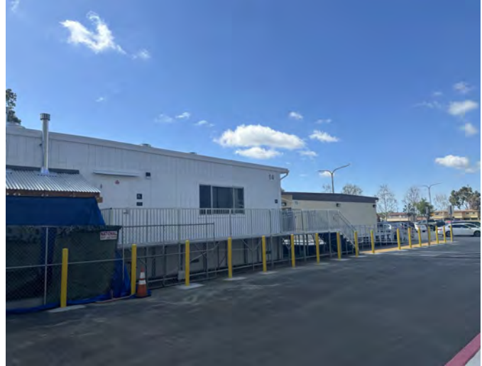
Swing Space—HRC Kitchen, Restroom and Dining Room — Modular Building Completed Construction
