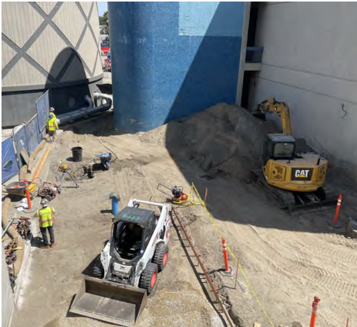
Fine Arts Building Renovation — Construction Activities
