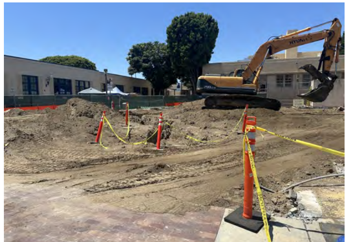
Wilshire Chiller Plant — Construction Activities
