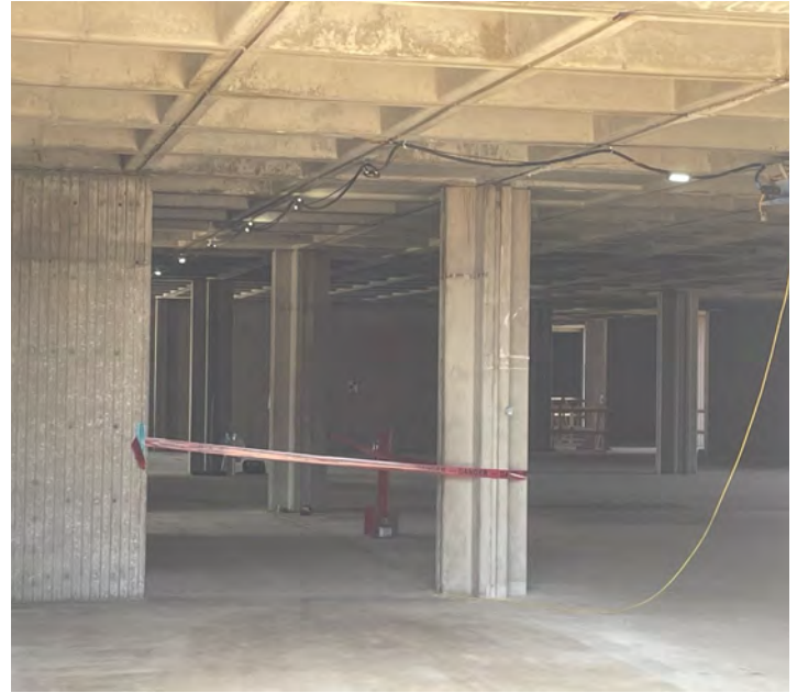
Fine Arts Building Renovation — Construction Activities
