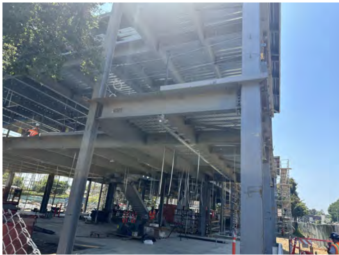
Chapman/Newell Instruction Building — Construction Activities
