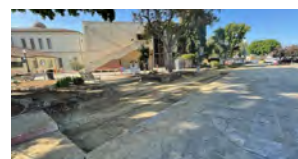
Renovate Building 300 [Construction]
