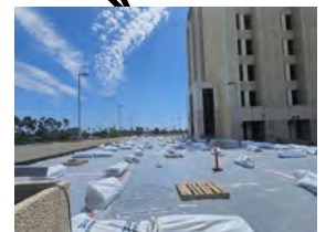
Anaheim Tower First Floor Life/Safety Renovation [Construction]
