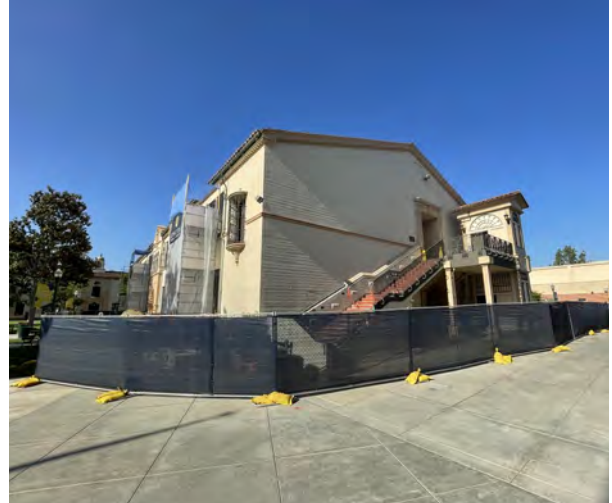
Renovate Building 300 - Construction Activities
