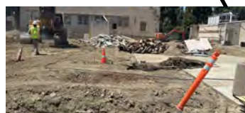
Wilshire Chiller Plant Relocation [Construction]
