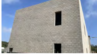
New Maintenance & Operations Building [Construction]
