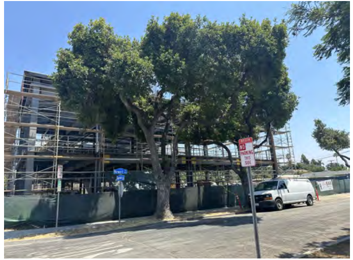
Chapman/Newell Instruction Building — Construction Activities
