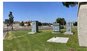
Electrical Vehicles (EV) SCE Charging Stations-Lot 4 [Construction]
