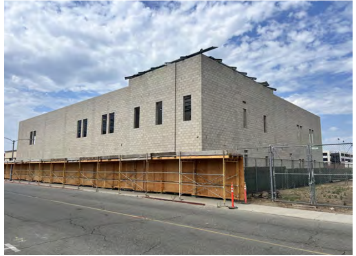
New M&O Building - Construction Activities
