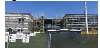
Chapman/Newell Instructional Building [Construction]
