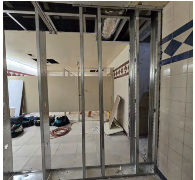
Anaheim Tower First Floor Life/Safety Renovation — Construction Activities
