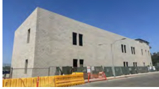
New Maintenance & Operations Building [Construction]
