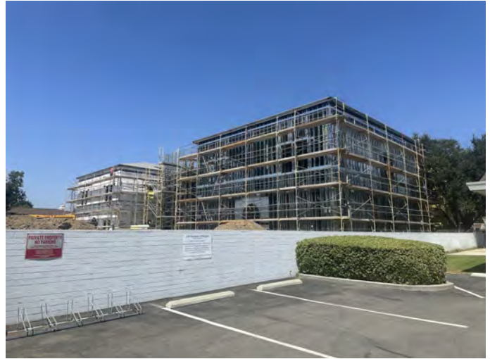
Chapman/Newell Instruction Building — Construction Activities
