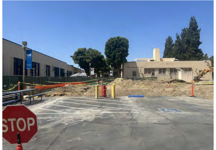
Wilshire Chiller Plant — Construction Activities
