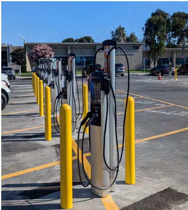
Electrical Vehicles (EV) SCE Charging Stations — Lot 4 — Construction Activities
