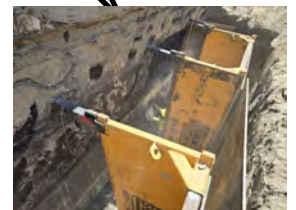
Anaheim Tower First Floor Life/ Safety Renovation [Construction]
