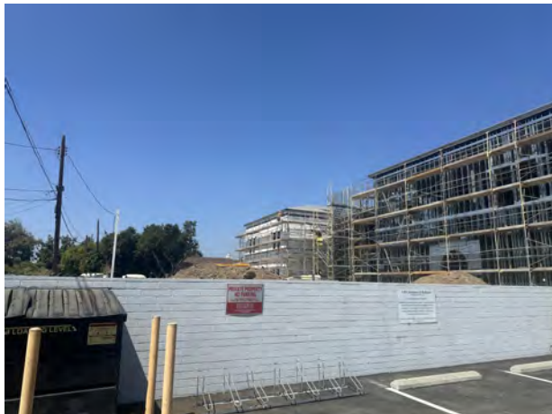
Chapman/Newell Instruction Building — Construction Activities
