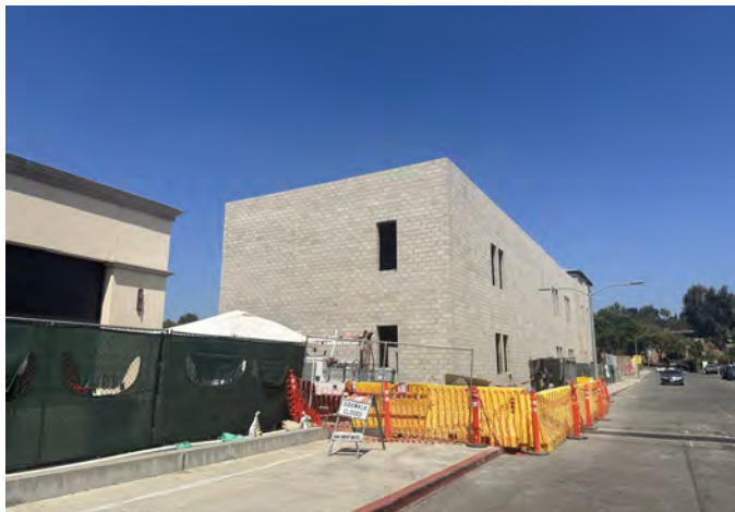
New M&O Building — Construction Activities
