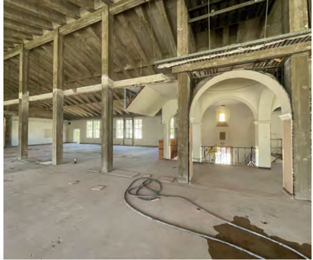
Renovate Building 300 - Construction Activities
