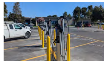
Electrical Vehicles (EV) SCE Charging Stations-Lot 4 [Construction]
