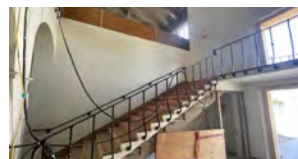
Renovate Building 300 [Construction]
