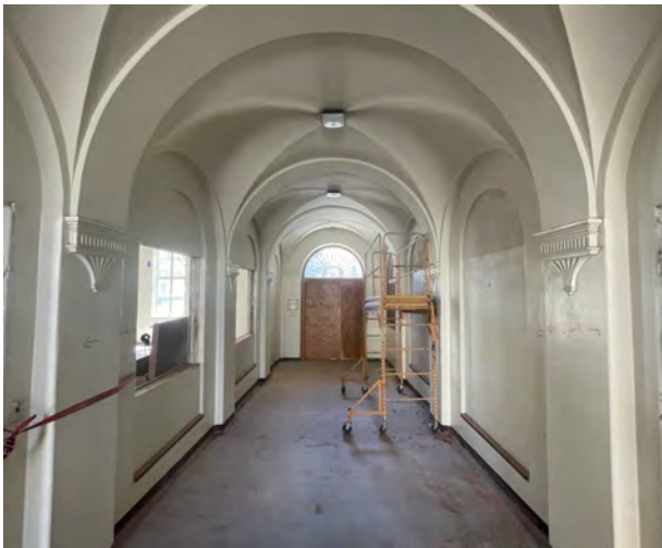
Renovate Building 300 - Construction Activities
