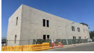
New Maintenance & Operations Building [Construction]
