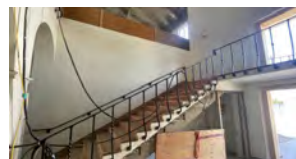
Renovate Building 300 [Construction]
