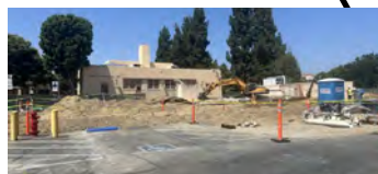
Wilshire Chiller Plant Relocation [Construction]
