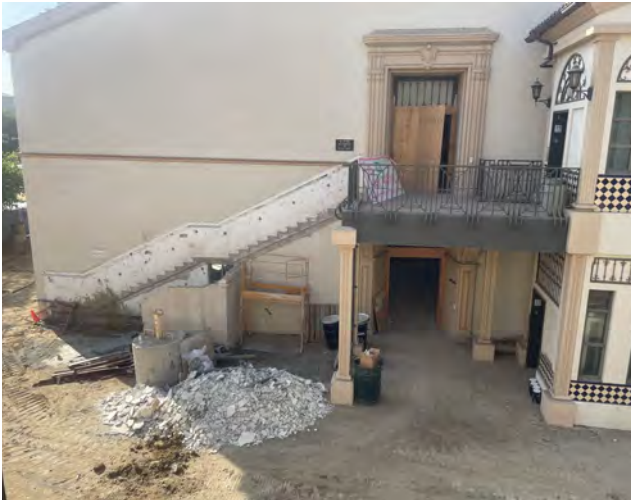
Renovate Building 300 - Stair Removal for CIDH and Pile Cap Installation
