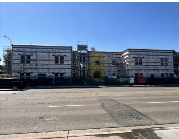
Chapman/Newell Instructional Building — Sheathing Placement and Building Envelope
