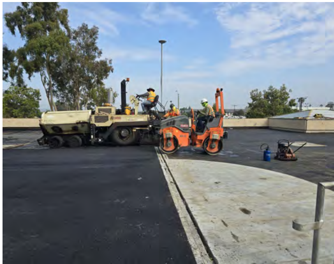
Anaheim Tower First Floor Life/Safety Renovation — Asphalt Layer Placement Activities
