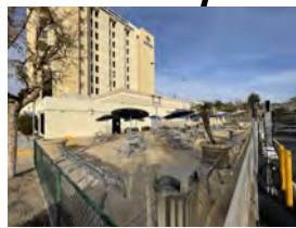
Outdoor Patio Remodel [Pre-Construction]
