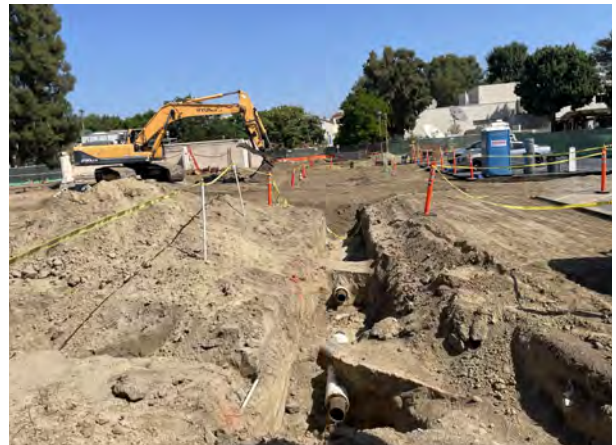
Wilshire Chiller Plant — Construction Activities
