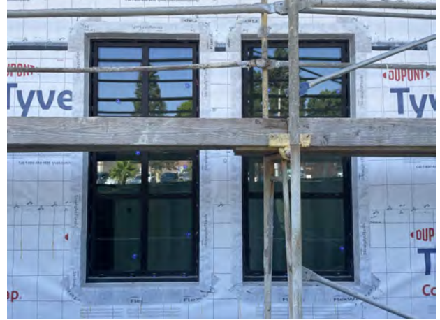
Chapman/Newell Instruction Building — Exterior View of Window Installation
