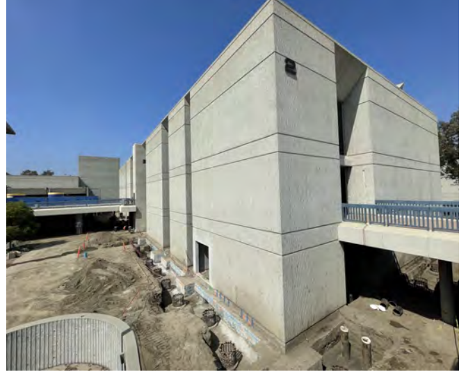
Fine Arts Building Renovation — Foundation Reinforcement Activities
