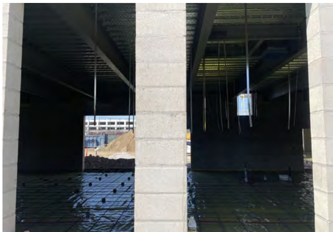
New M&O Building — Preparation for Slab-on-Grade Concrete Pouring
