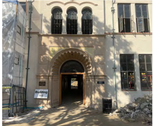
Renovate Building 300 - Construction Activities
