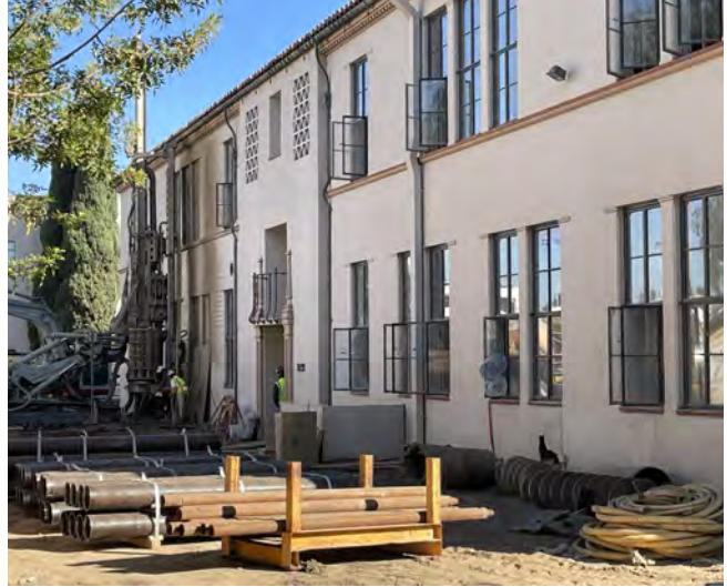
Renovate Building 300 - Construction Activities
