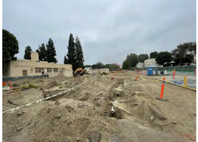
Wilshire Chiller Plant Relocation — Construction Activities
