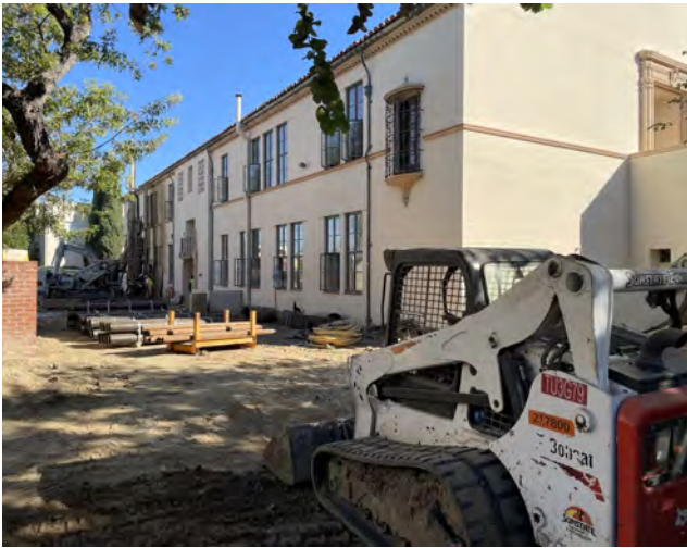
Renovate Building 300 - Construction Activities
