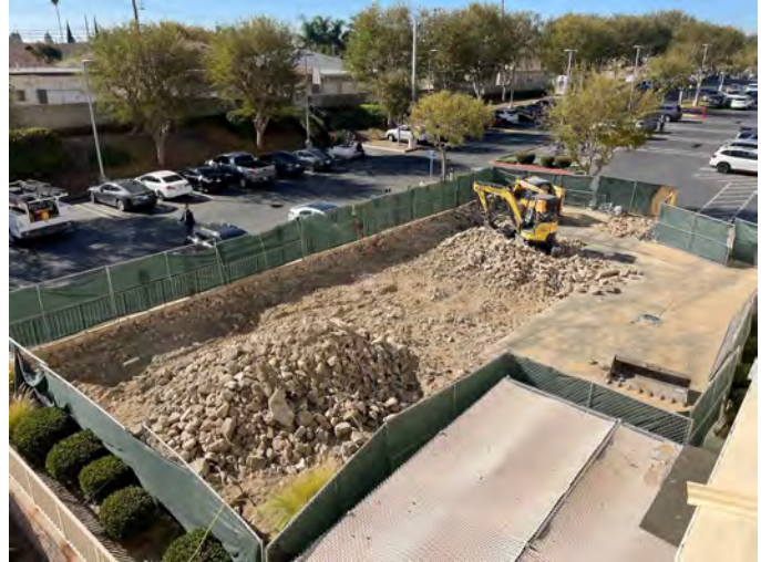
Outdoor Patio Remodel — Construction Activities
