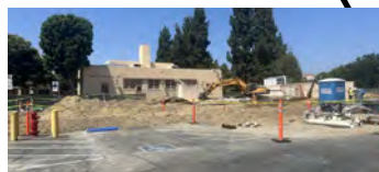
Wilshire Chiller Plant Relocation [Construction]
