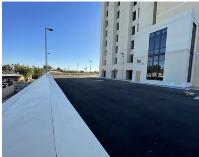
Anaheim Tower First Floor Life/Safety Renovation — Construction Activities
