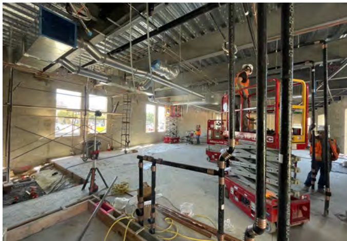
New M&O Building — Construction Activities
