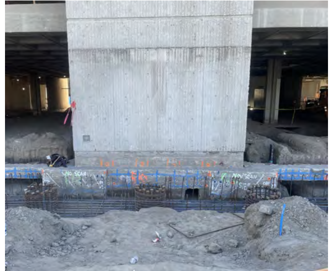
Fine Arts Building Renovation — Foundation Reinforcement Activities
