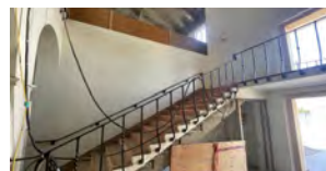
Renovate Building 300 [Construction]
