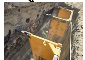
Anaheim Tower First Floor Life/Safety Renovation [Construction]
