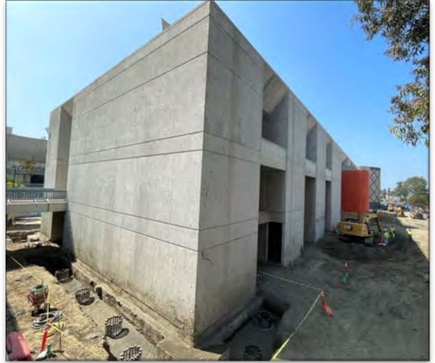
Fine Arts Building Renovation — Construction Activities
