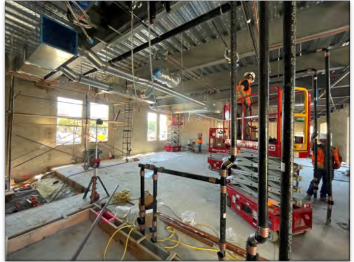
New M&O Building—Construction Activities
