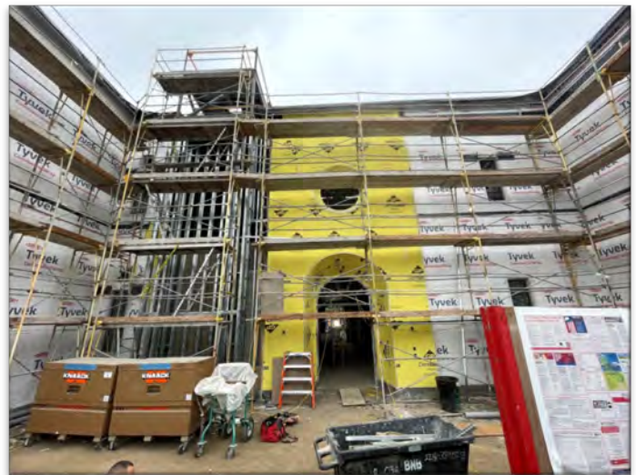
Chapman/Newell Instructional Building—Construction Activities
