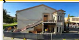
Renovate Building 300 [Construction]
