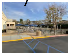
Outdoor Patio Remodel [Construction]
