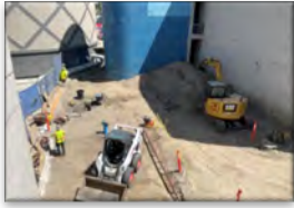
Fine Arts Building Renovation [Construction]
