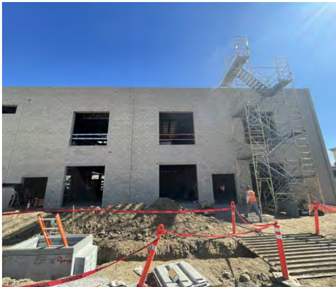
New M&O Building -- Construction Activities
