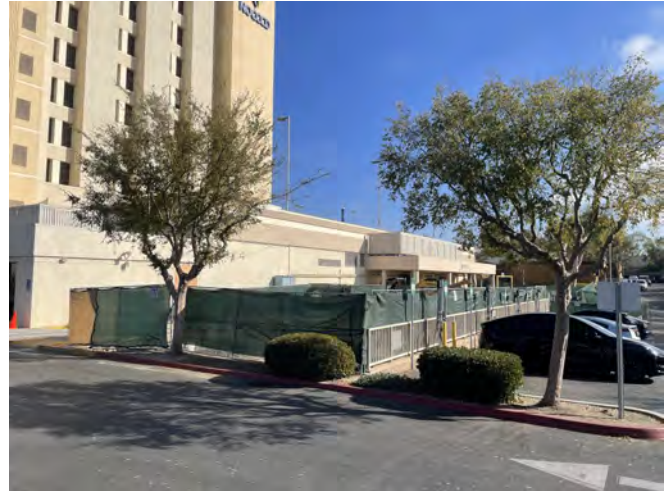
Outdoor Patio Remodel: Construction Activities
