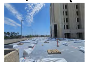
Anaheim Tower First Floor Life/Safety Renovation [Construction]
