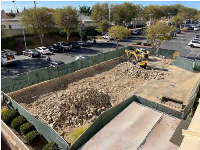
Outdoor Patio Remodel: Construction Activities
