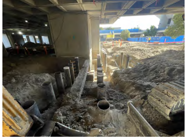
Fine Arts Building Renovation — Steel Pile Driving Activities
