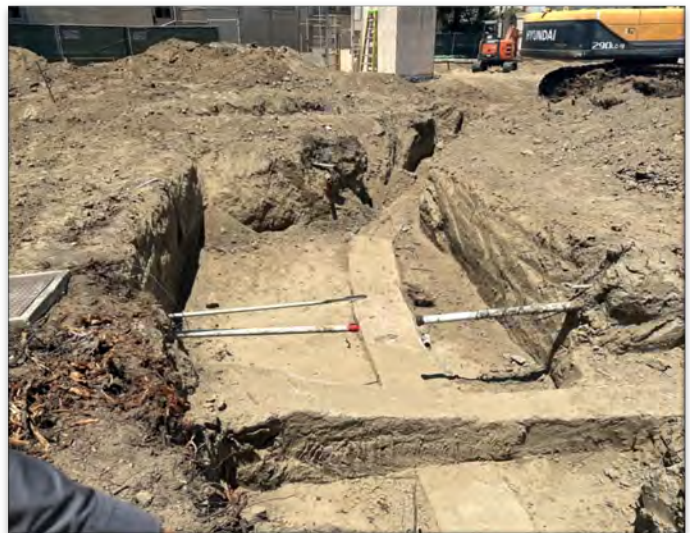
Wilshire Chiller Plant Relocation—Construction Activities
