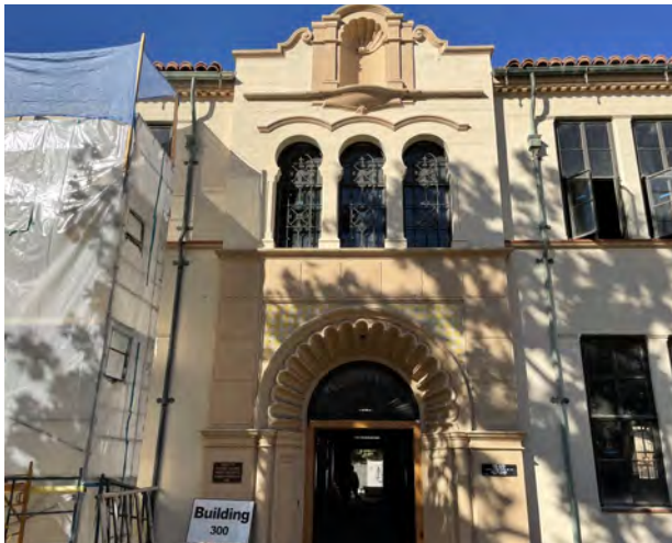
Renovate Building 300 - Construction Activities
