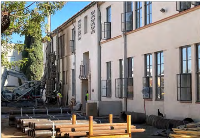
Renovate Building 300 - Construction Activities
