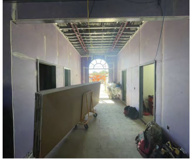
Chapman/Newell Instructional Building -- Construction Activities
