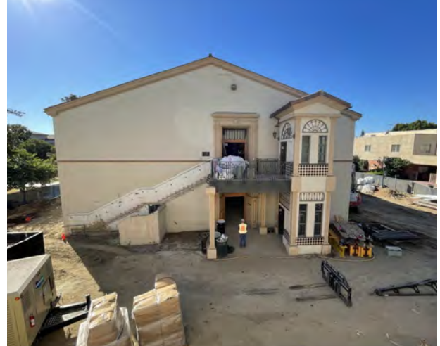
Renovate Building 300 - Construction Activities
