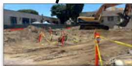
Wilshire Chiller Plant Relocation [Construction]
