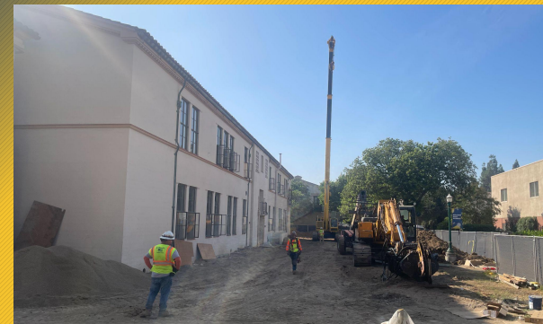
CIDH Pile Drilling Activities
