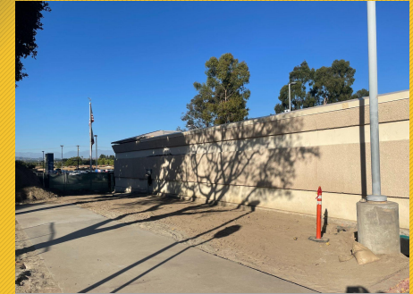
Completed Retaining Wall
