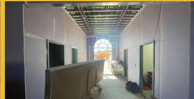
Interior Drywall Placement
