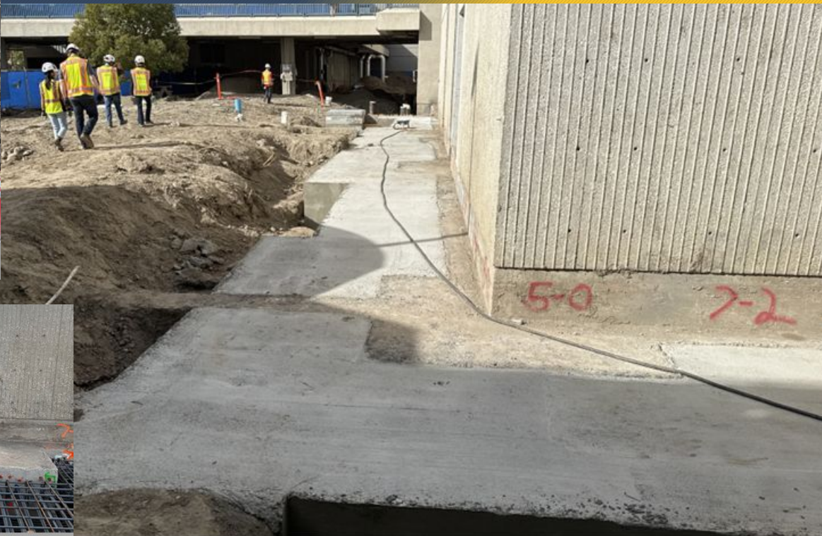
Completed Pile Cap at Southeast Corner
