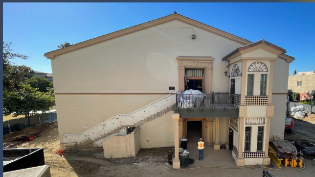
Demolished Stairwell for CIDH Drilling
