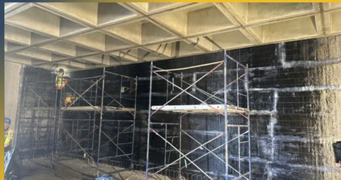
Fiber Reinforced Polymer (FRP) Installation
