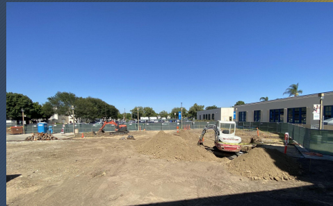
Building Foundation Site Excavation
