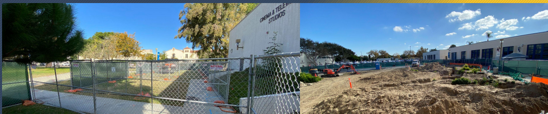
New Fence Line Placement and Excavation for Unforeseen Condition Rerouting
