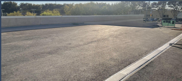
Asphalt Paving and Expansion Joint Completed
