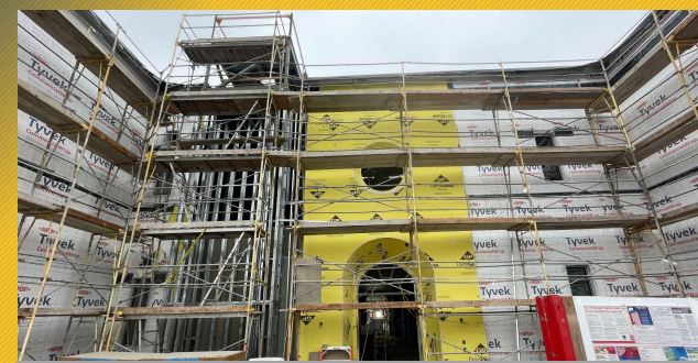
Building Envelope and Sheathing Activities
