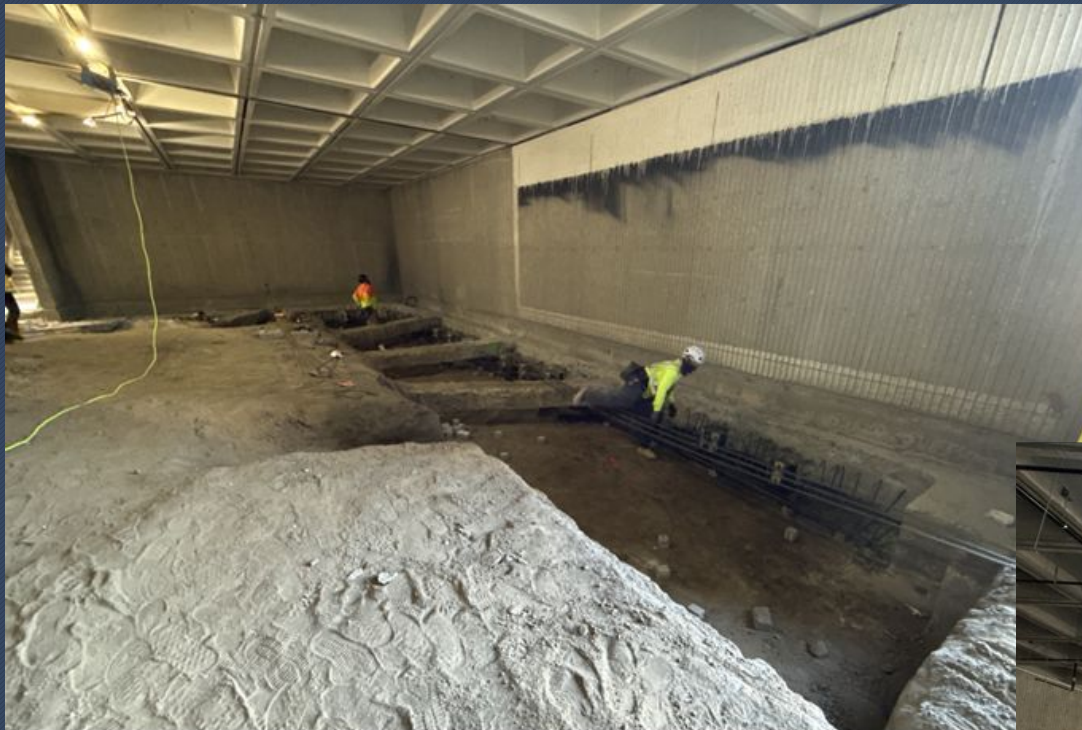
Interior Rebar Placement for Pile Cap
