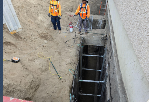
West Retaining Wall Activities
