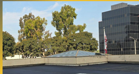
Flower Bed Roofing Activities
