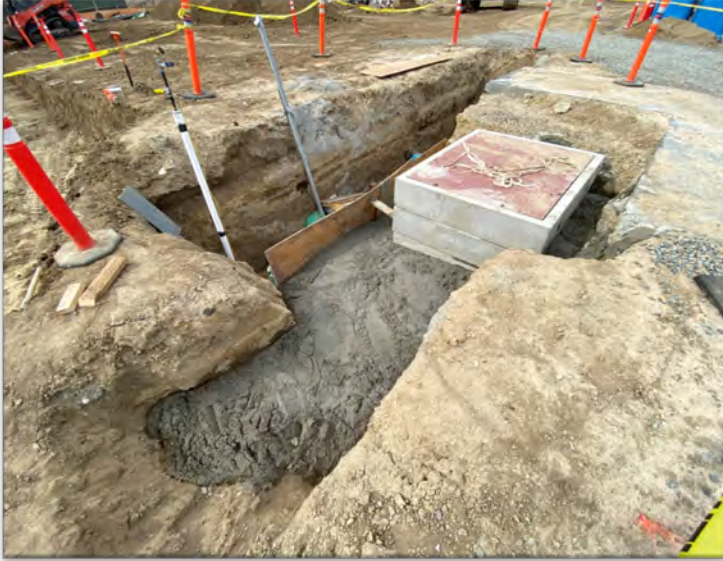
Wilshire Chiller Plant Relocation — Vault Backfilling Activities
