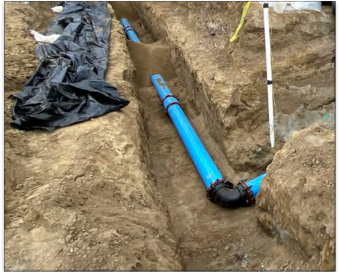
Wilshire Chiller Plant Relocation — Fire Hydrant Line Reroute
