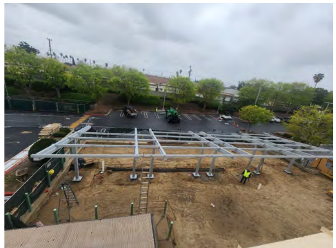
Outdoor Patio Remodel — Shade Structure Installation
