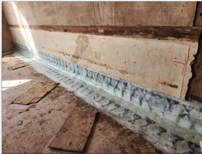
Renovate Building 300 — First Floor Fiber Reinforced Polymer Application
