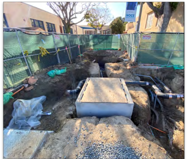
Wilshire Chiller Plant Relocation — Vault Placement Activities
