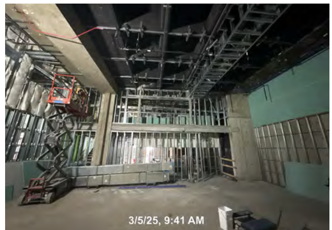
Fine Arts Building Renovation — Wall Framing and Rough-in Activities
