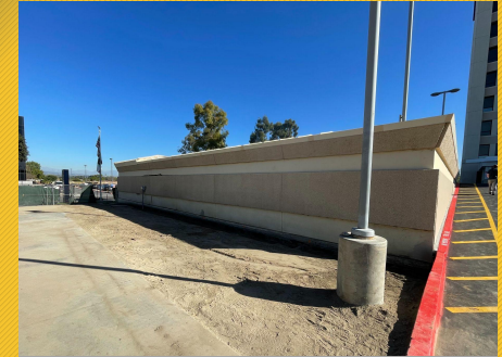
Completed Retaining Wall
