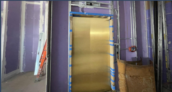
Elevator Installation Activities
