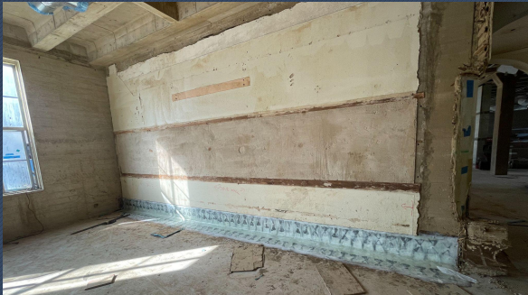
First-Floor FRP Application
