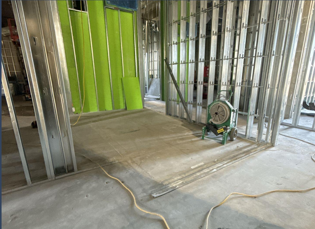
Interior Metal Wall Framing
