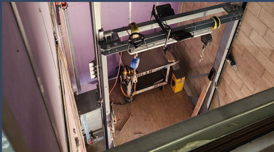
Elevator Installation Activities
