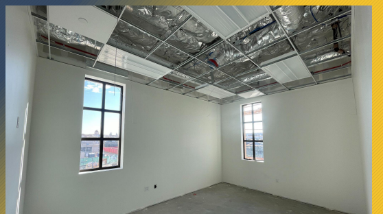
Interior Painting Activities
