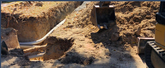
Trenching, Conduit, Electrical Vault Placement and Slurry
