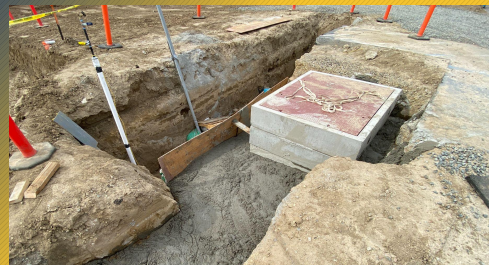
Trenching, Conduit, Electrical Vault Placement and Slurry
