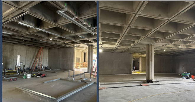
Completed Concrete Pours
