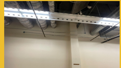
Water Intrusion Repairs Completed
