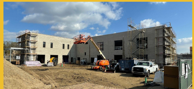
Exterior Facade Activities
