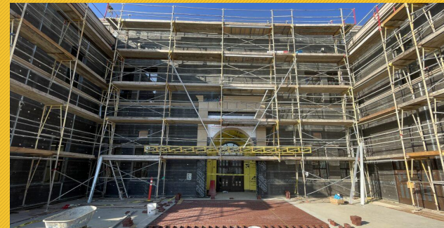
Building Envelope and Facade Activities
