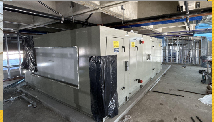
Air Handler Unit Installation
