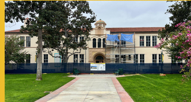
Building Facade and Window Restoration
