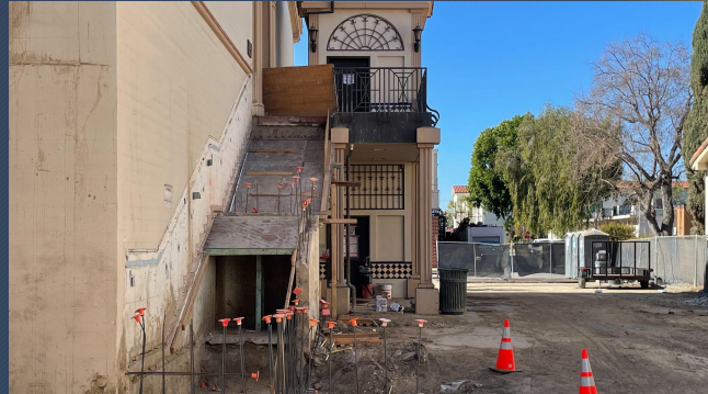
Stairwell Reconstruction after Pile Drilling
