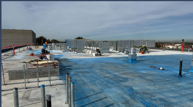
Waterproofing on Roof
