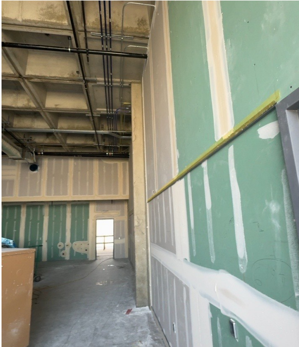
Fine Arts Building Renovation — Drywall Installation
