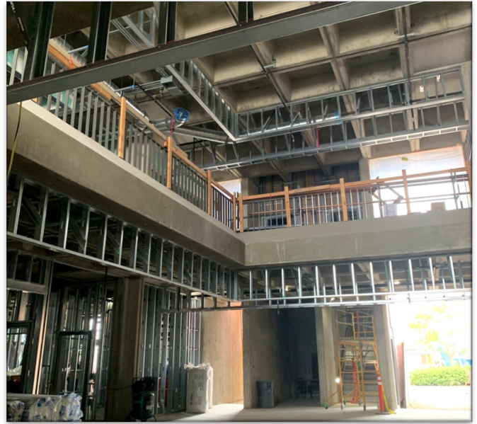
Fine Arts Building Renovation — Metal Stud Wall Framing
