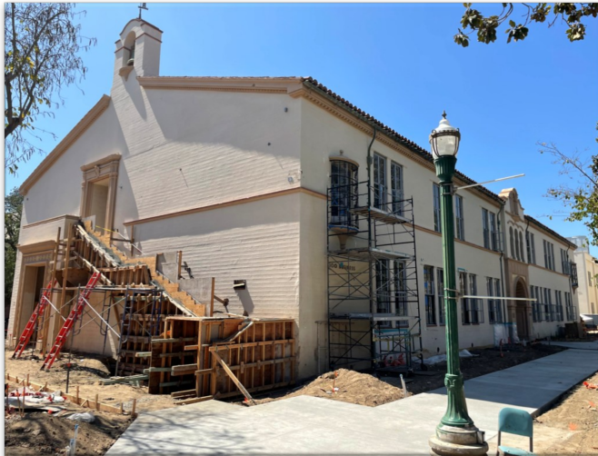
Renovate Building 300 — South Stair Restoration
