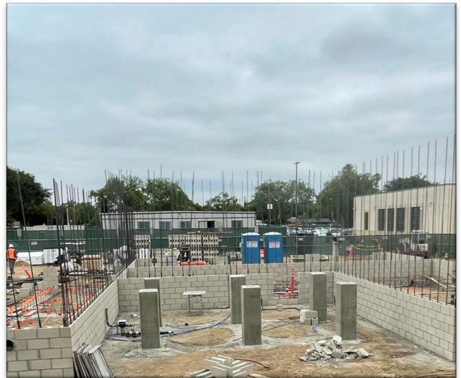
Wilshire Chiller Plant Relocation — CMU Wall Installation and Finished Grade Beam
