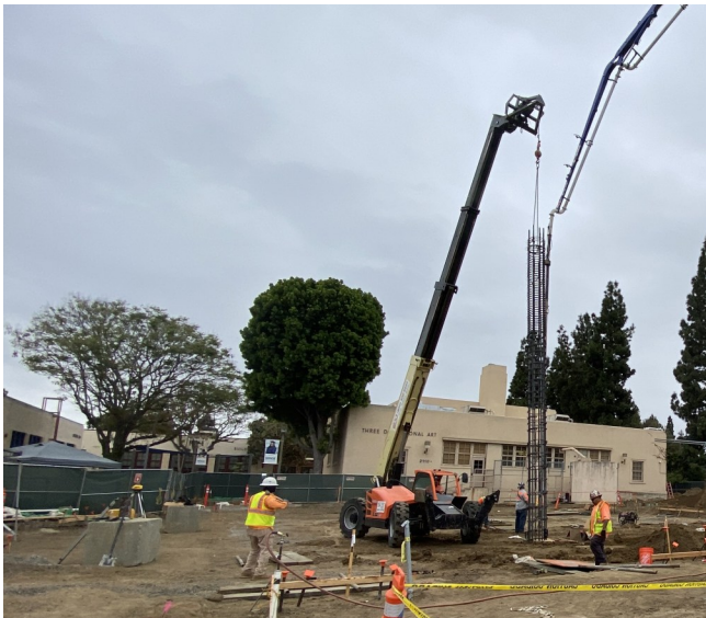
Wilshire Chiller Plant Relocation — Reinforcement Bar Cage Placement for Pile Drilling
