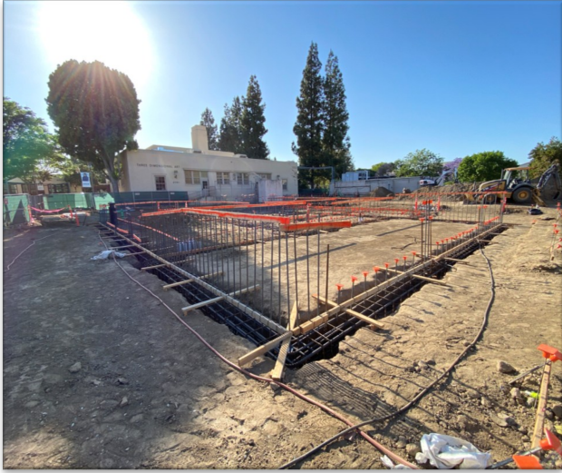
Wilshire Chiller Plant Relocation — Reinforcement Bar Placement for Grade Beam Foundation
