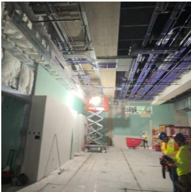
Fine Arts Building Renovation — Insulation and Overhead Mechanical, Electrical, and Plumbing Installation
