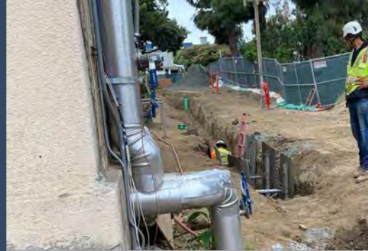
Sewer Line Trenching and Placement
