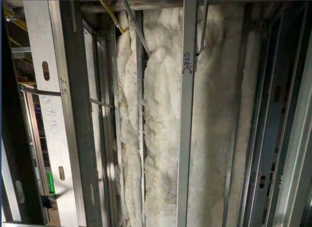
In-Wall Insulation Application
