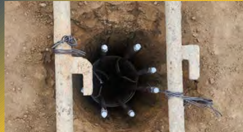
Cast-in-Drill-Hole-Pile Drilling Activities
