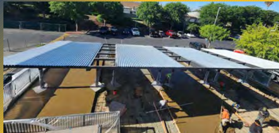
Sheet Metal Placement and Concrete Pours for Slab on Grade
