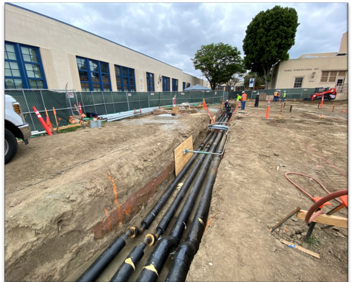
Wilshire Chiller Plant Relocation — Underground Piping Installation
