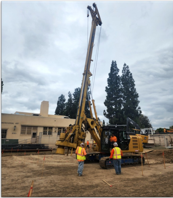
Wilshire Chiller Plant Relocation — Pile Drilling Activities
