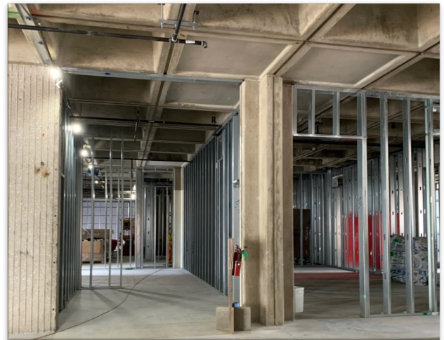
Fine Arts Building Renovation — Wall Framing
