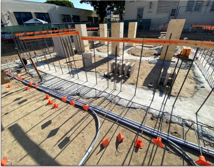
Wilshire Chiller Plant Relocation — Completed Grade Beams and Concrete Masonry Wall Installation
