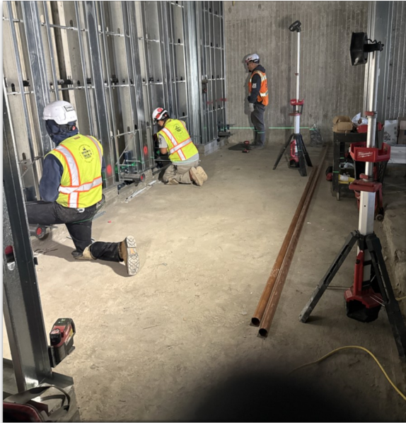
Fine Arts Building Renovation — Wall Framing
