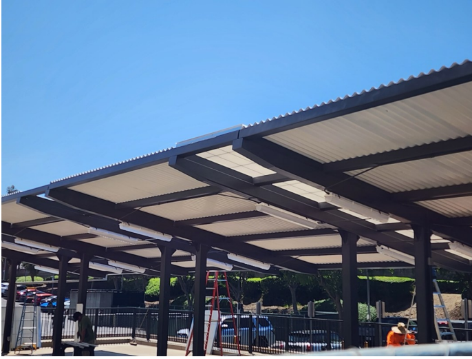
Outdoor Patio Remodel — Installed Translucent Kalwall Panels
