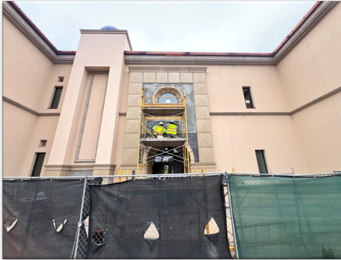
Student Support Center — Building Façade Ornamental Tile Placement
