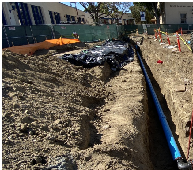
Wilshire Chiller Plant Relocation — Fire Hydrant Water Line Reroute
