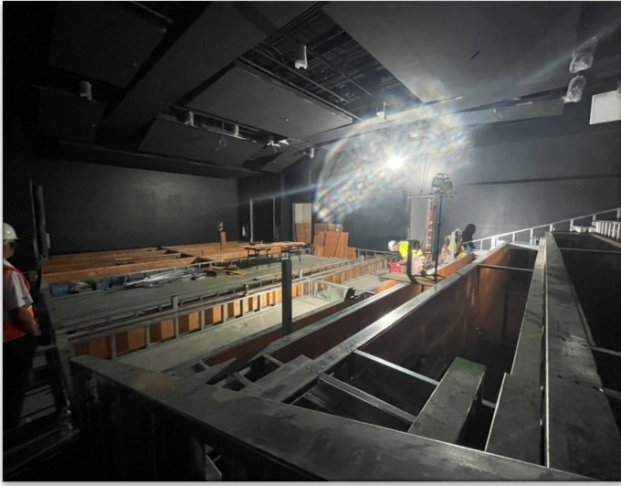
Fine Arts Building Renovation — Recital Hall Stage and Theater Seating Construction
