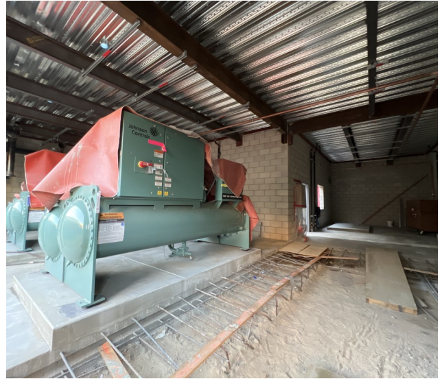
Wilshire Chiller Plant Relocation — Steel Roof Decking Installation; Completed CMU Walls, and Equipment Placement on Mechanical Pad
