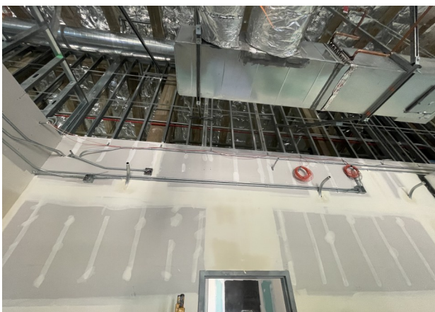
Renovate Building 300 — Drywall and Mechanical, Electrical, and Plumbing Installed
