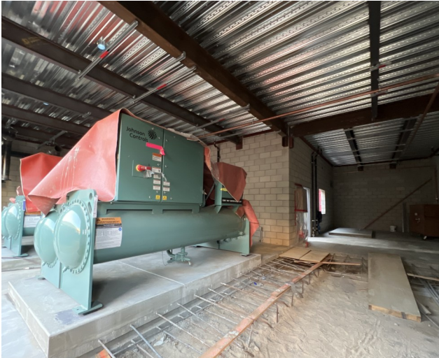
Wilshire Chiller Plant Relocation — Steel Roof Decking Installation; Completed CMU Walls, and Equipment Placement on Mechanical Pad
