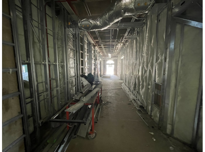
Renovate Building 300 — Walls Framed and Insulated
