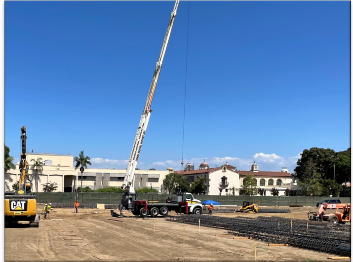
New Performing Arts Complex — Cast-In-Drill-Hole Activities
