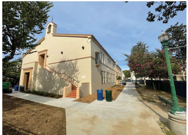
Renovate Building 300 South Stairs
