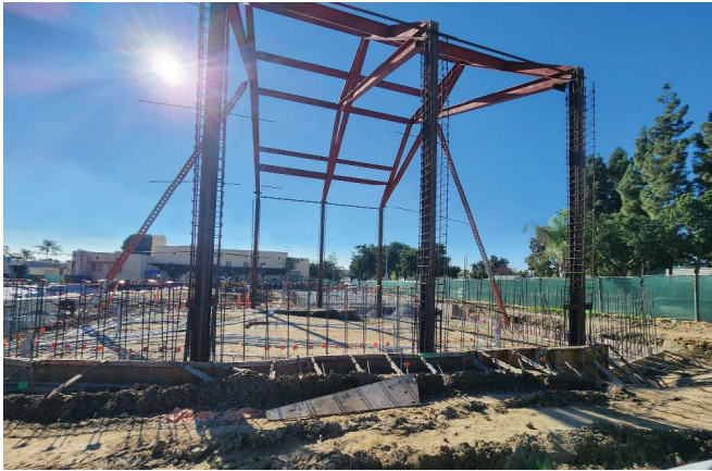
New Performing Arts Complex Steel Structure in West Building Recital Hall
