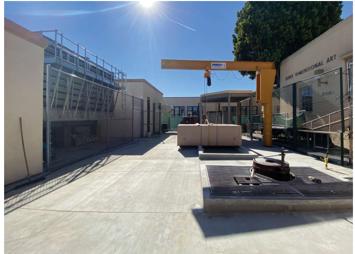
Wilshire Chiller Plant Relocation Jib Crane in Place in Art Yard
