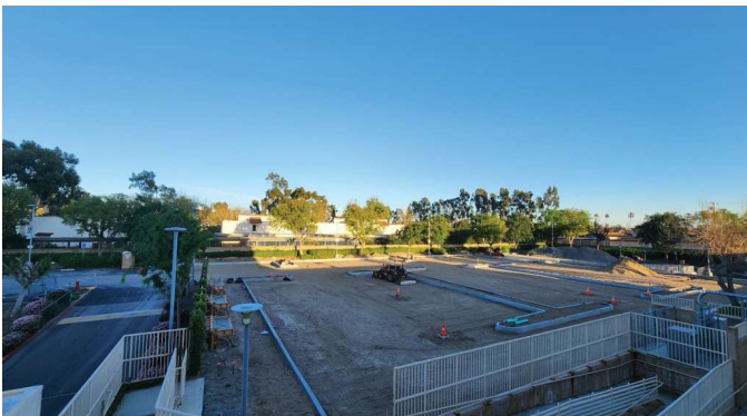
Restore East Parking Lot Completed Grading and Concrete Curb Work
