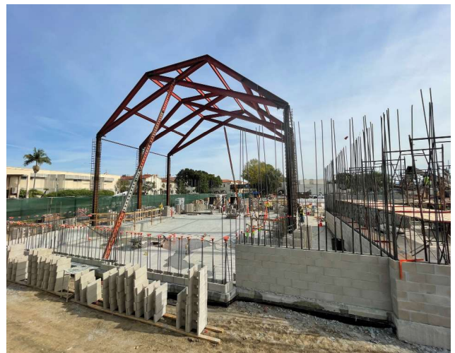
New Performing Arts Complex Concrete Masonry Unit Installation
