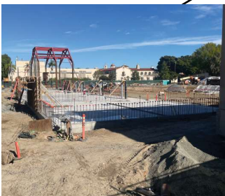
New Performing Arts Complex - Demolish Buildings 1100 and 1300 [Construction]
