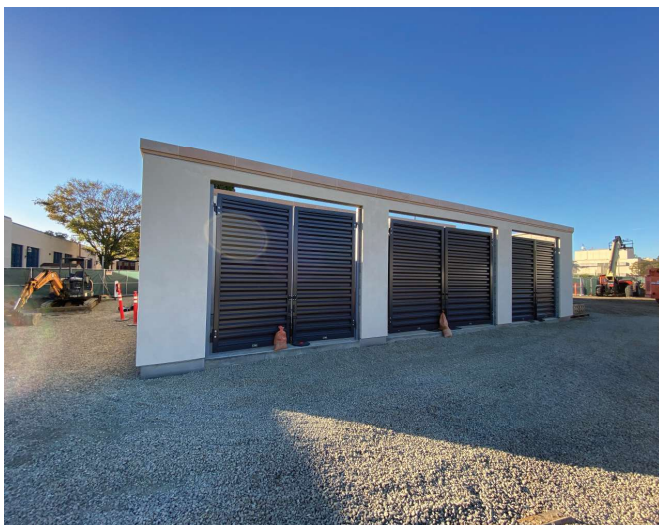
Wilshire Chiller Plant Relocation Completed SCE Yard
