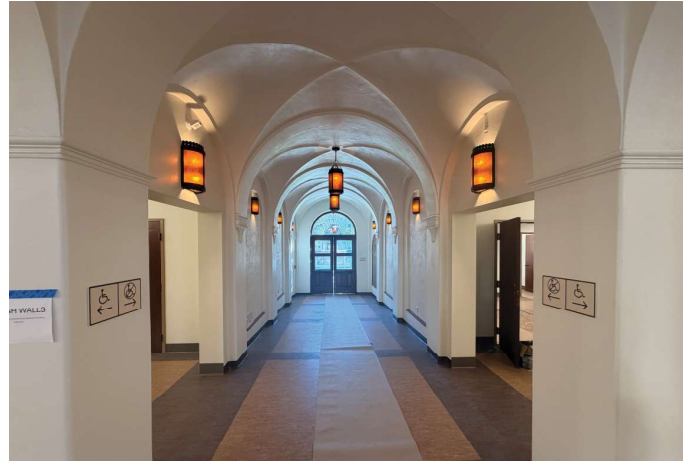
Renovate Building 300 Completed Flooring
