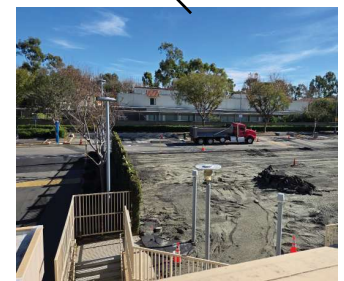
Restore East Parking Lot [Construction]
