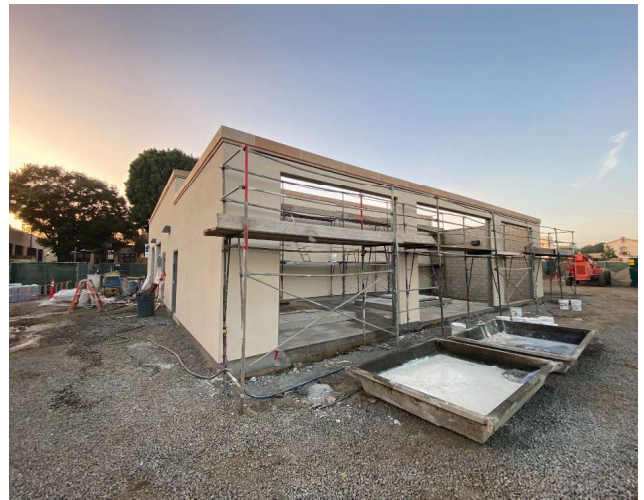
Wilshire Chiller Plant Relocation SCE Electrical Yard Wall Plastering
