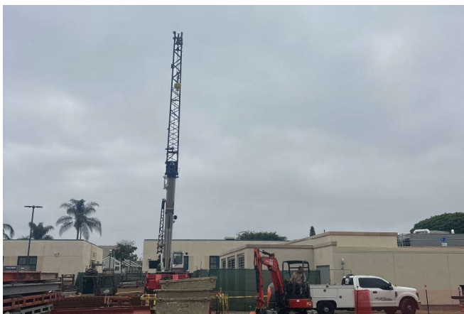
New Performing Arts Complex Preparations for Cast-In-Drill Hole Upcoming in mid-May
