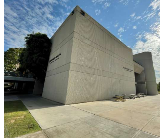
SEM (FASS) Building 3 Demolition and Site Restoration [Upcoming Planning]
