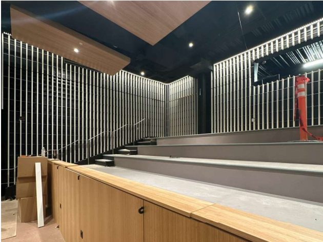
Fine Arts Building Renovation Wood Slat Installation
