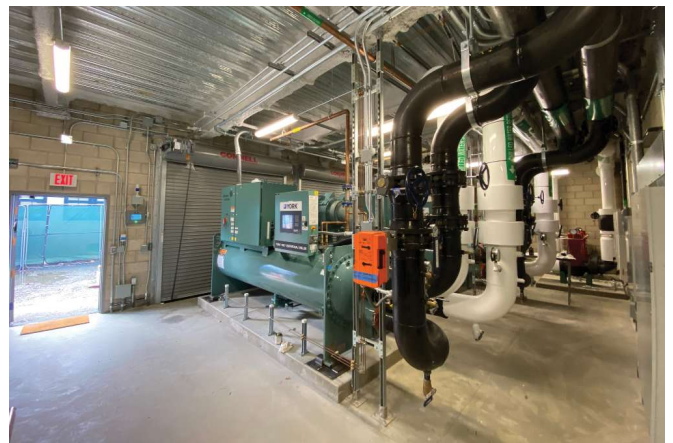
Wilshire Chiller Plant Relocation Completed Site
