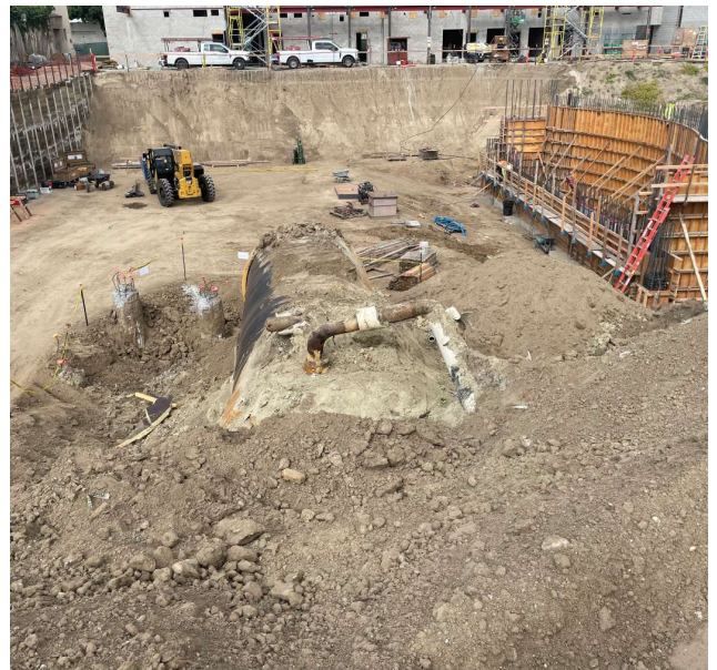
New Performing Arts Complex 30,000-Gallon Tank Testing and Removal
