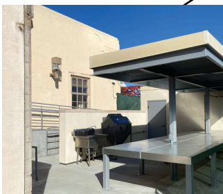
Wilshire Chiller Plant Relocation [Close-Out]
