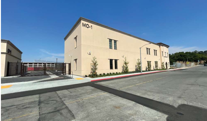
New Maintenance & Operations Completed Project
