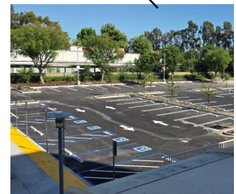
Restore East Parking Lot [Close-Out]
