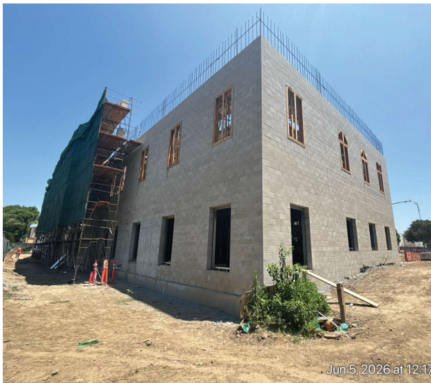
New Performing Arts Complex West Building CMU Wall Installation
