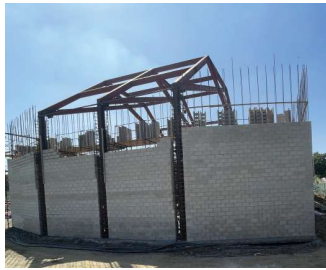
New Performing Arts Complex - Demolish Buildings 1100 and 1300 [Construction]
