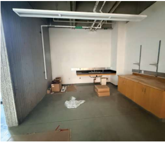
Fine Arts Renovation [Construction]
