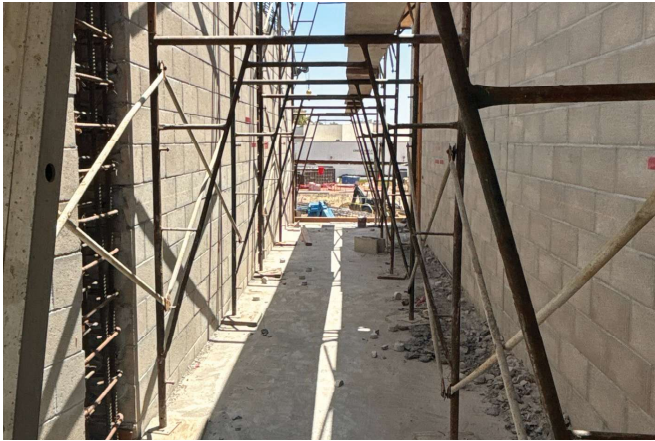
New Performing Arts Complex West Building In-Wall Rough-In Activities
