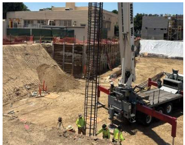
New Performing Arts Complex Caisson Drilling in Orchestra Pit
