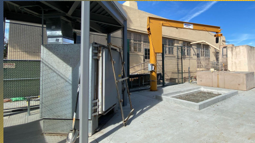
Kiln Furnace and Canopy and Jib Crane
