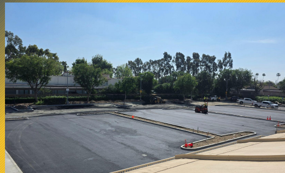
Leveling and Asphalt Paving
