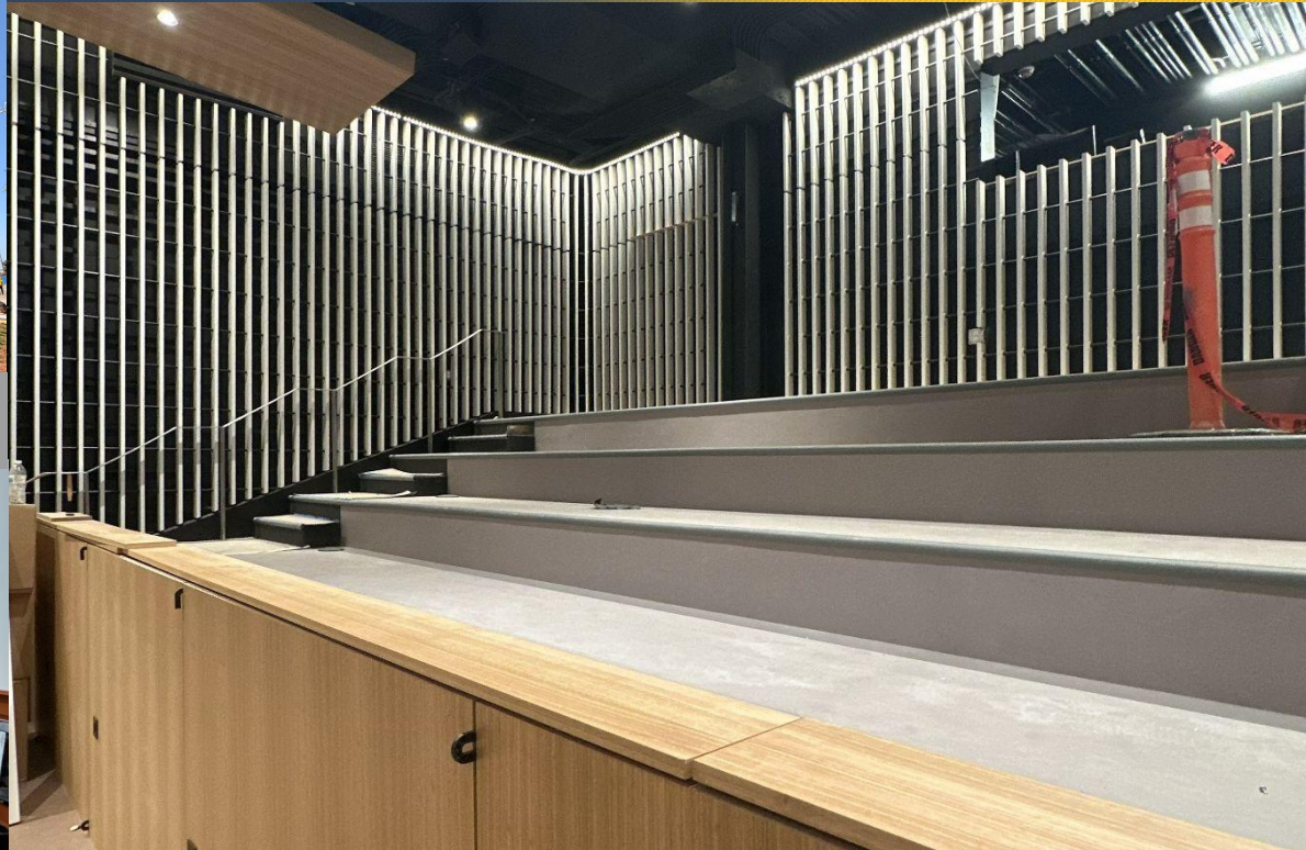
Wood Slat Installation at Third Floor Recital Hall
