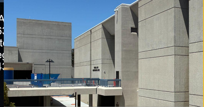
Seismic Guardrail Retrofit
