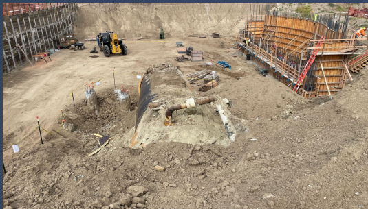
Unforeseen Condition - 30K-Gallon Tank Removal, Excavation in Orchestra Pit, and Cast-In-Drill-Hole Work
