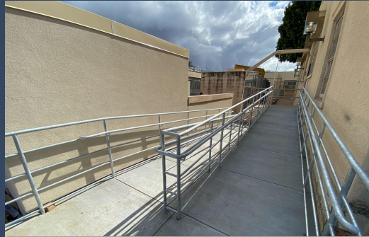
Completed Accessibility Ramp
