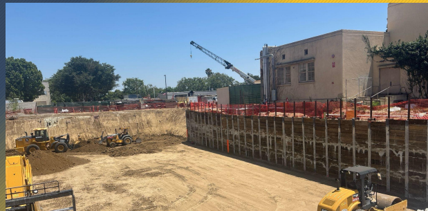
Unforeseen Condition - 30K-Gallon Tank Removal, Excavation in Orchestra Pit, and Cast-In-Drill-Hole Work
