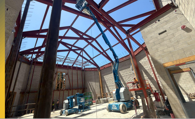
West Building Activities: Steel Decking and CMU Wall Installation
