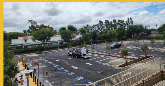
EV Charging Station Installation
