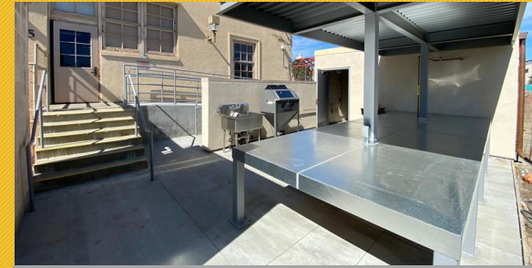
Workbench with Table Surface Installed at Art Yard
