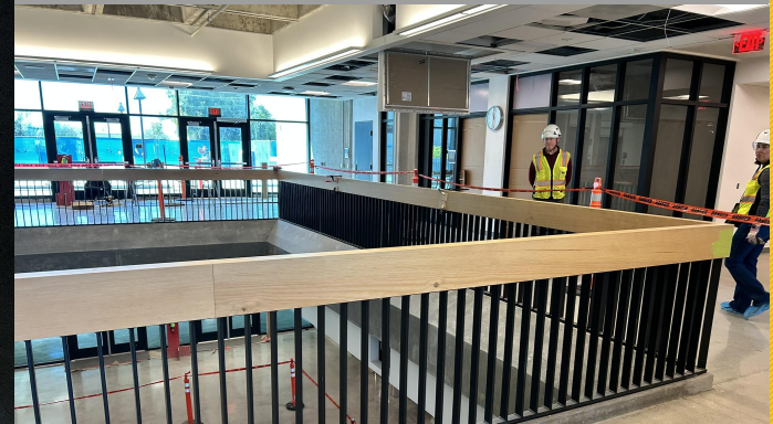
Mezzanine Lobby Handrail Activities
