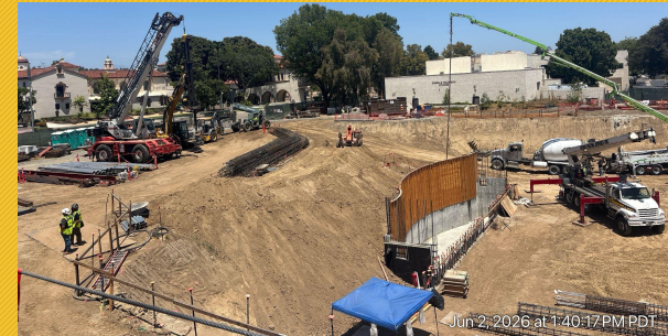
Unforeseen Condition - 30K-Gallon Tank Removal, Excavation in Orchestra Pit, and Cast-In-Drill-Hole Work
