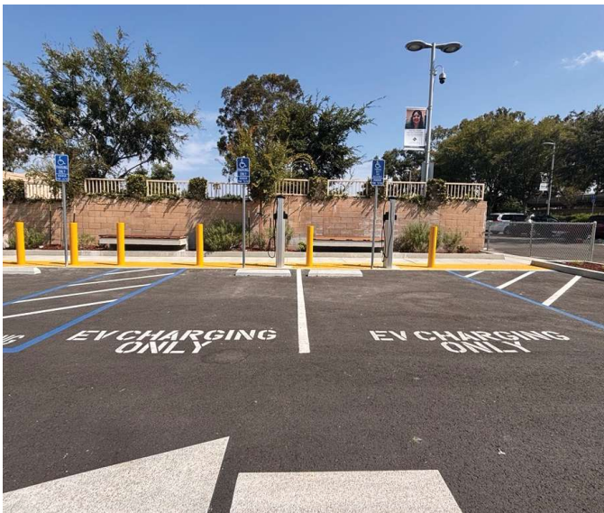
Restore East Parking Lot Completed Parking Lot, Including ADA Accessible EV Charging Stations
