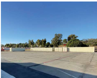
Swing Space - New M&O [Dismantling]
