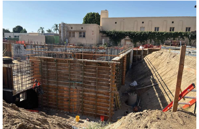
New Performing Arts Complex Main Building Basement Concrete Wall Erection
