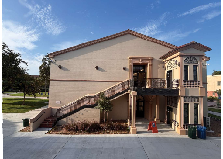
Renovate Building 300 Completed Stairs on the North end of the Building
