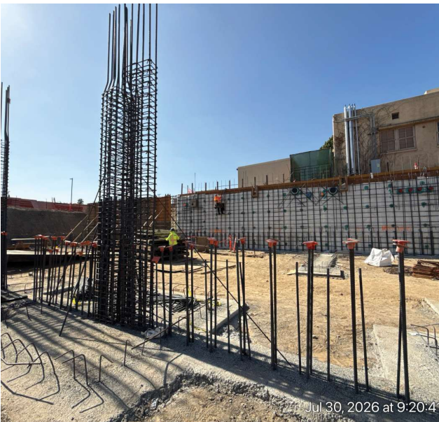
New Performing Arts Complex Basement Foundation Work at Main Building
