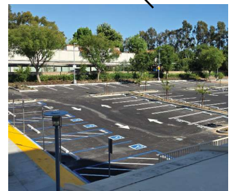
Restore East Parking Lot [Close-Out]
