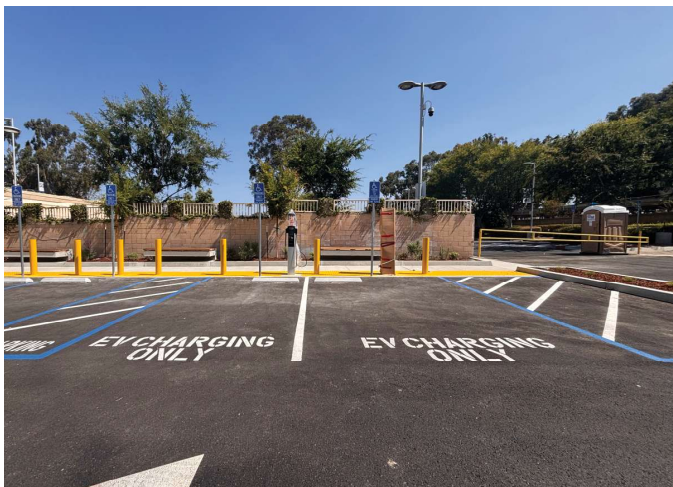
Restore East Parking Lot Installed Electrical Vehicle Charging Stations at ADA Parking Stalls
