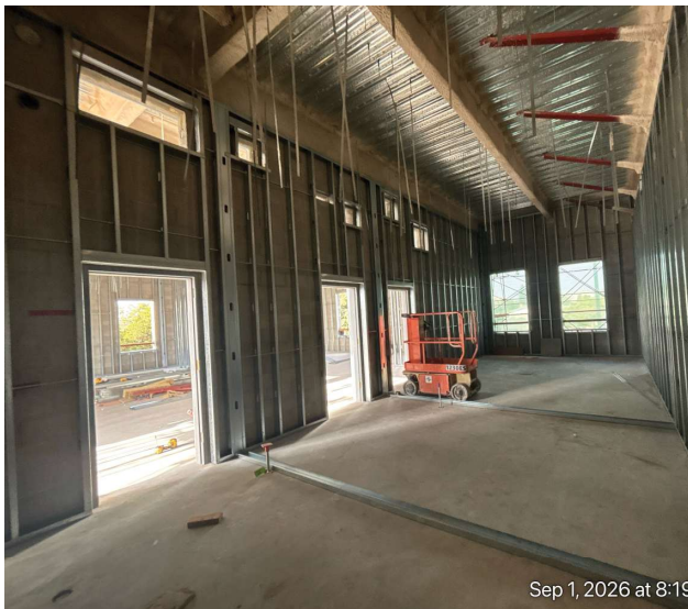
New Performing Arts Complex West Building Metal Stud Framing
