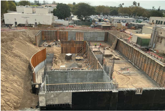
New Performing Arts Complex Basement Concrete Wall Pours and Orchestra Pit Development
