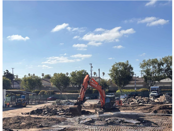
Exterior Green Community Space Enhancement Site Demolition
