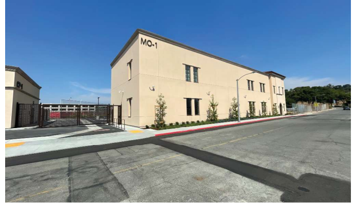
New Maintenance & Operations Building Completed Project
